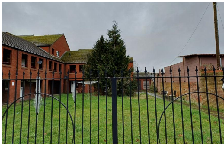
Relationship of ground level at flats to application site
