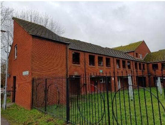
Flats to the south-west viewed from rear on Avon Place
