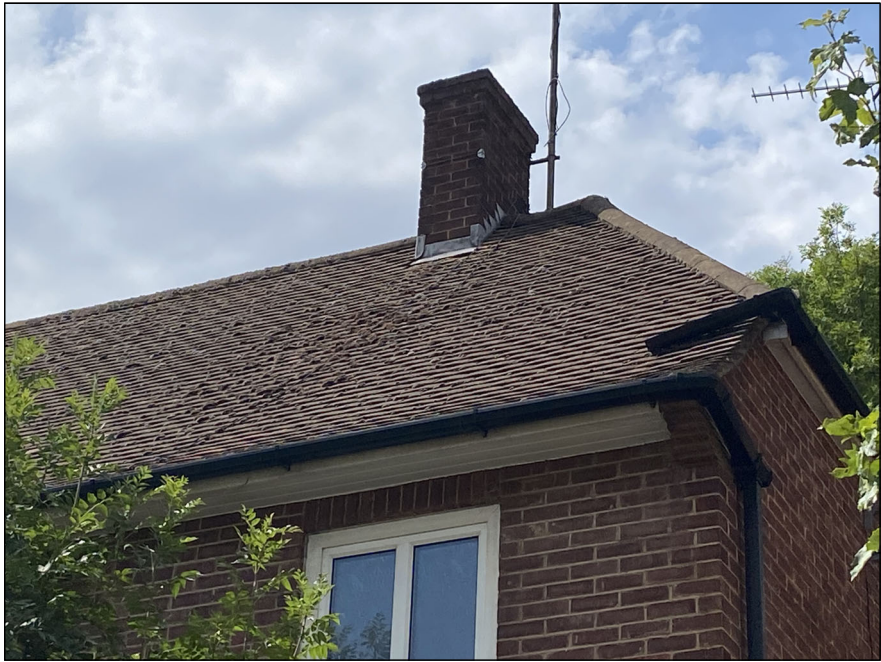
Photograph 2: Showing the front elevation of the house.
