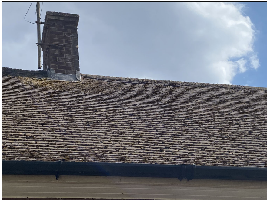
Photograph 3: Showing the roof which was in good condition and well-sealed.
