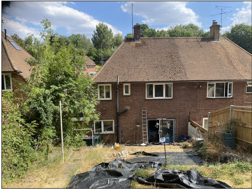
Photograph 1: Showing the rear elevation of the house.
