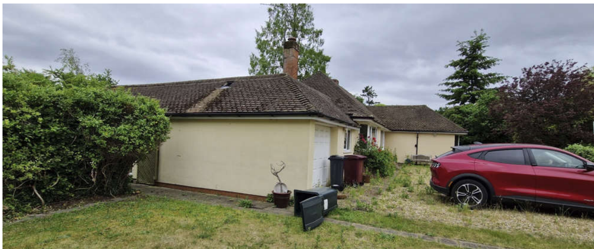
Image 3: View of existing front/side elevation showing the existing lower roof above the garage and annexe room
