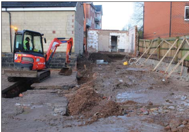
Plate 1. Flat 1, looking West
