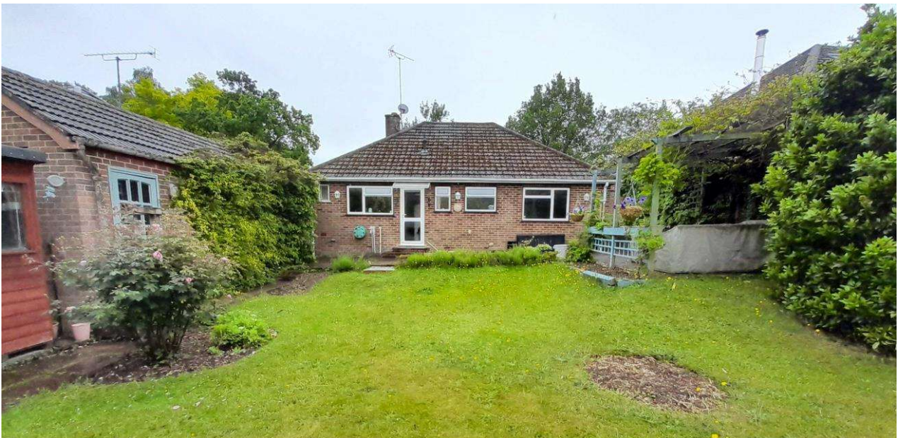
Looking towards existing (north facing) rear elevation with garage on left of picture and no.20 neighbour to the left
