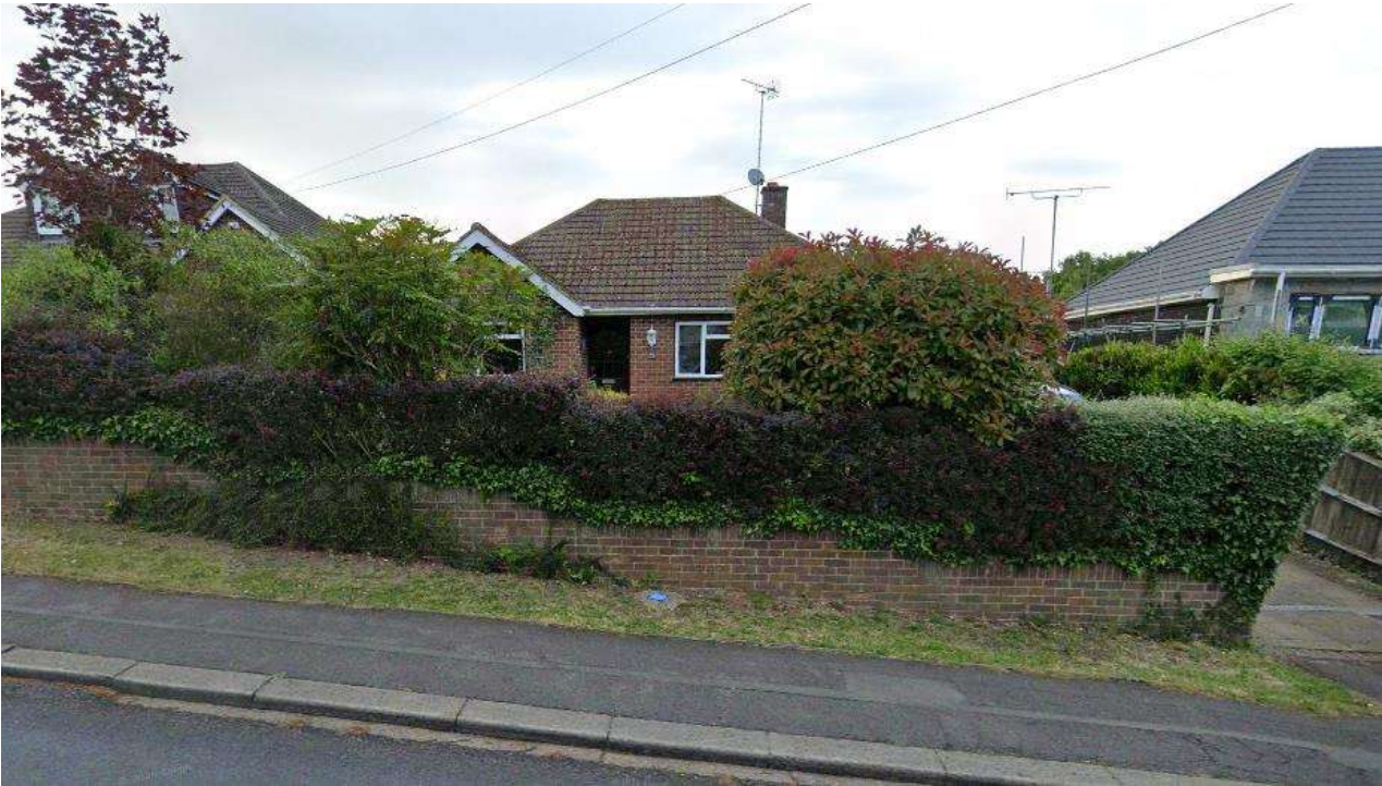
Looking towards existing (south facing) front elevation
