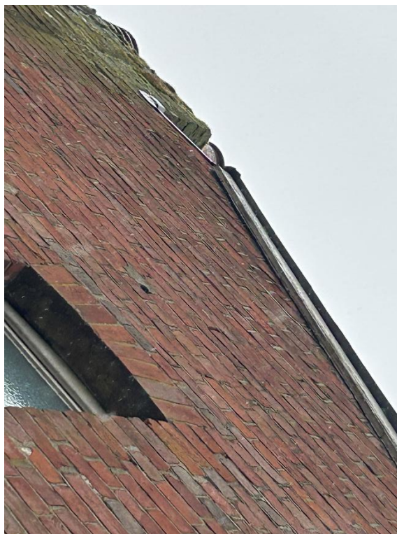
Photograph 8: Flashing and fascia board
