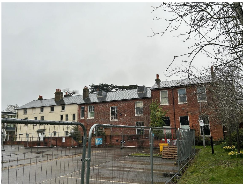
Photograph 5: B1 Southern elevation
