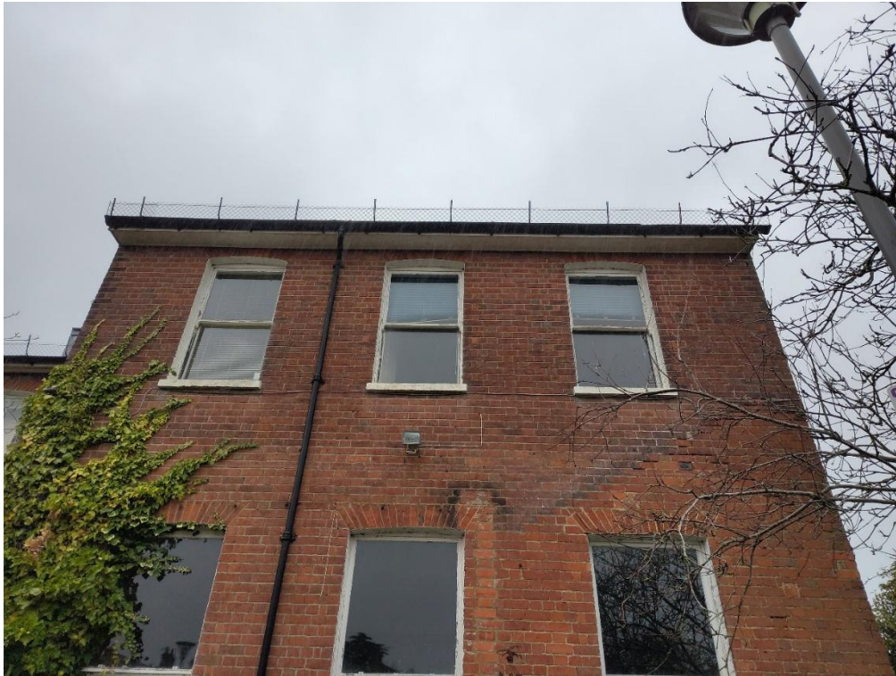
Photograph 6: Soffit Boxes on B1
