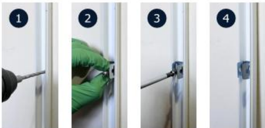
D Clip installation sequence
