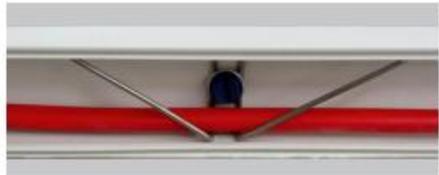
Cable held with Firefly clips
