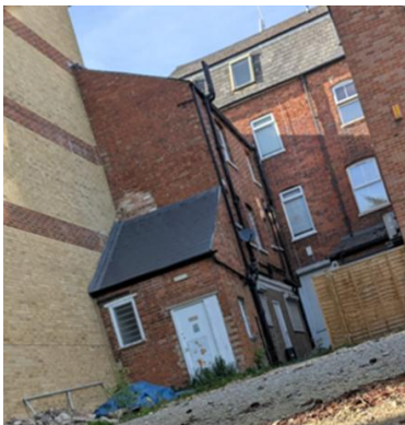
Figure 2: 29 April 26 site rear photo
