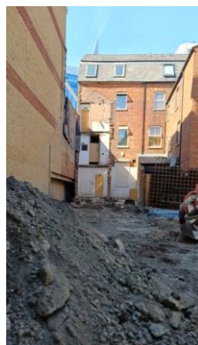
Figure 3: 7 July 2026 site rear photo
