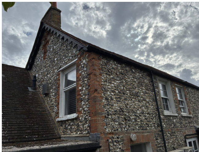
Figure 2 Window NE-1 in Context of Building
