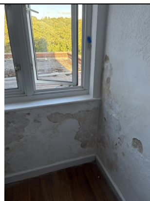
Figure 4 Internal damp
