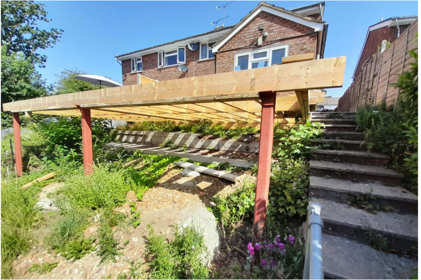
Looking north towards host property rear elevation, steps and handrail and unauthorised decking
