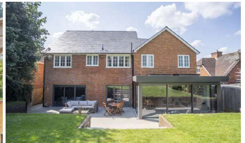
Residential extension using vertical cladding and large glazed openings to distinguish new additions from the original dwelling.
