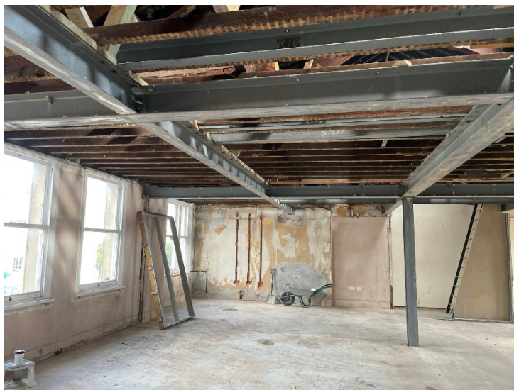
The second floor interior to be converted
