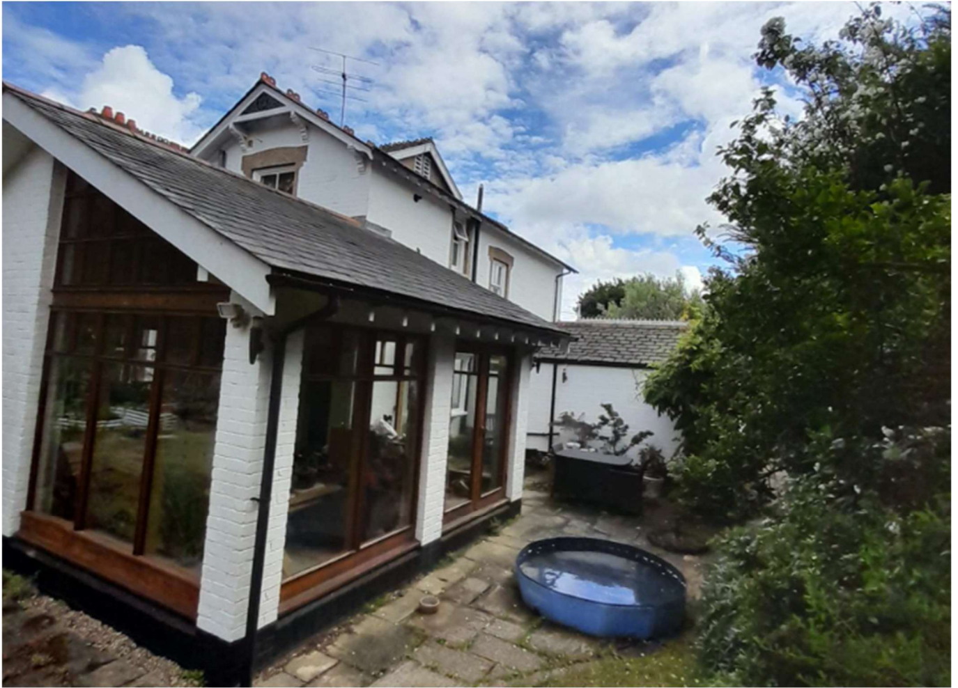
Side elevation looking southeast, existing tiled utility roof in view
