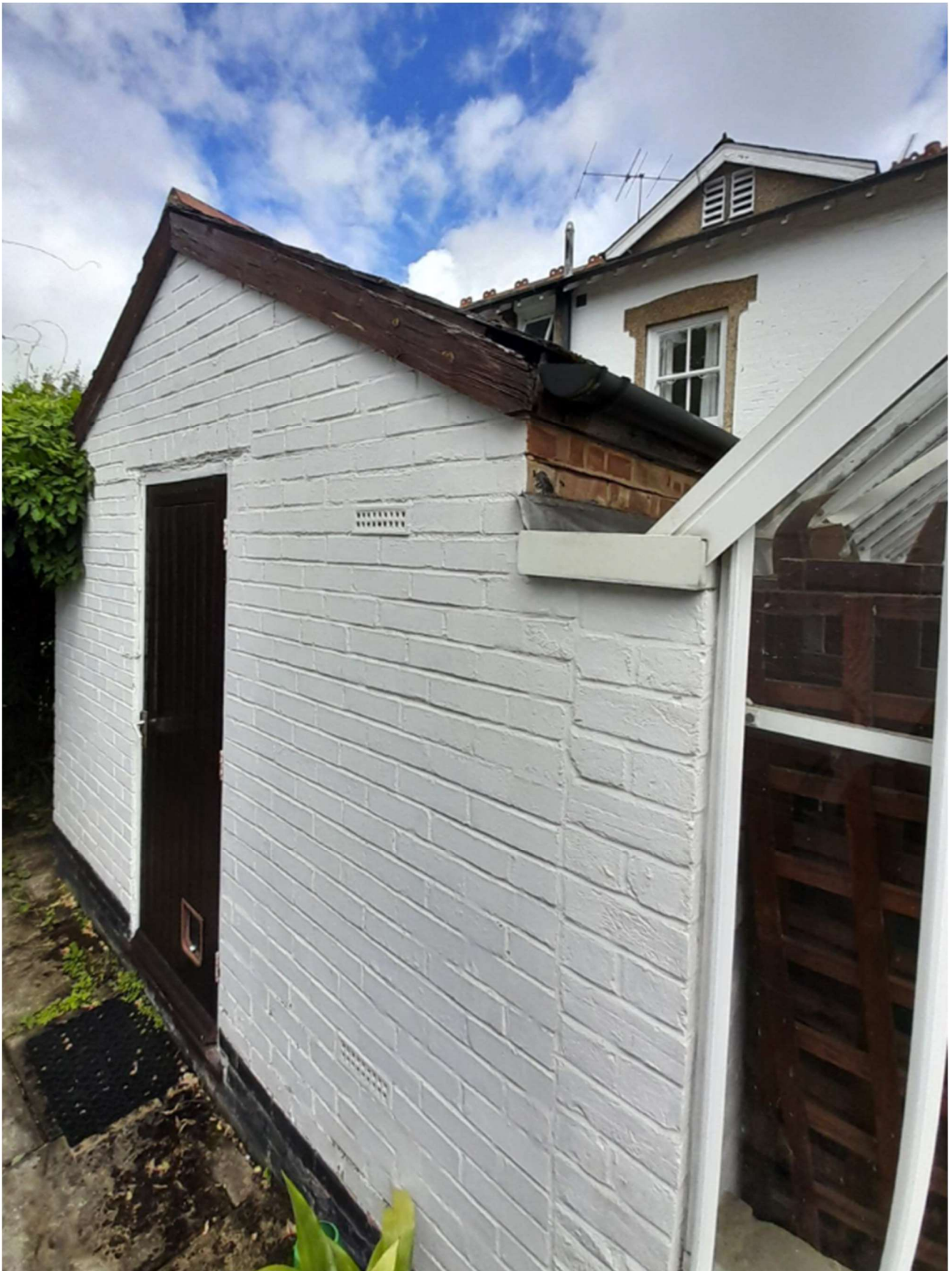
Side elevation of existing utility room
