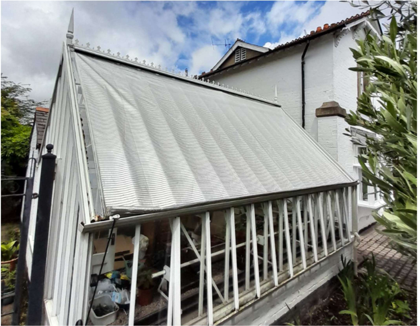
Front elevation looking northeast
