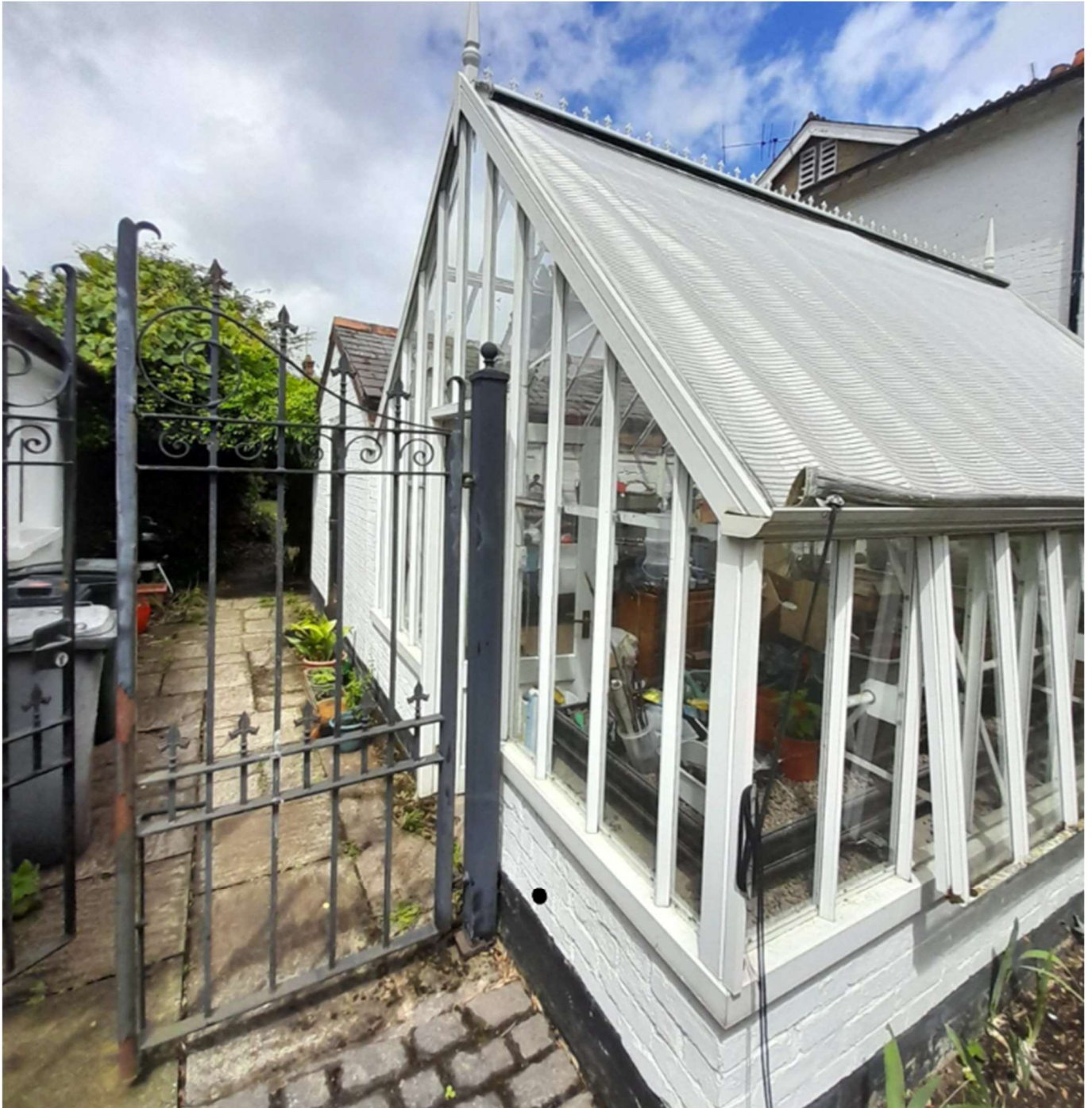
Existing side elevation with tiled roof of existing utility room just in shot
