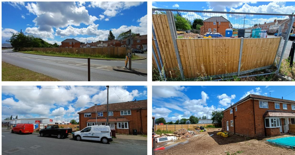
Figure 1 - Site visit photos - 9 June 2026
