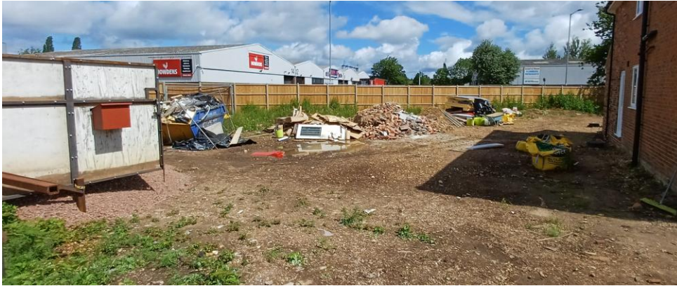
Figure 6 - Water pooling during site visit
