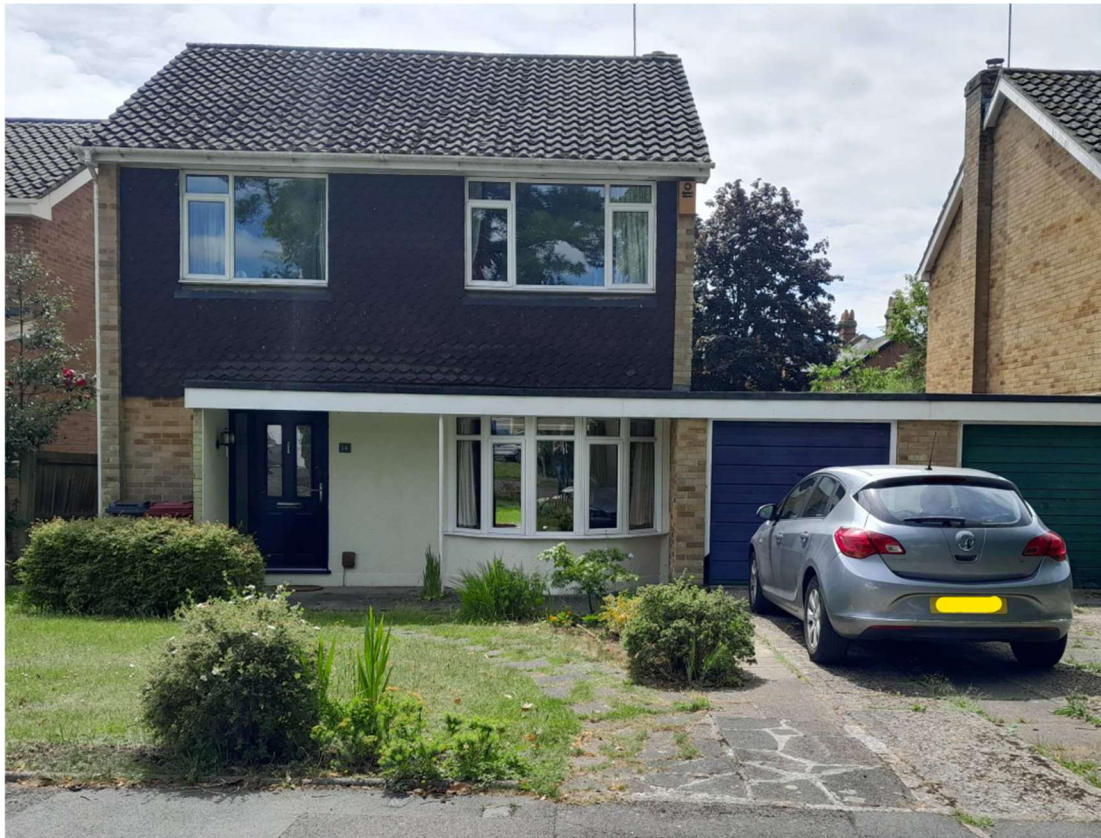
Looking towards the existing front elevation
