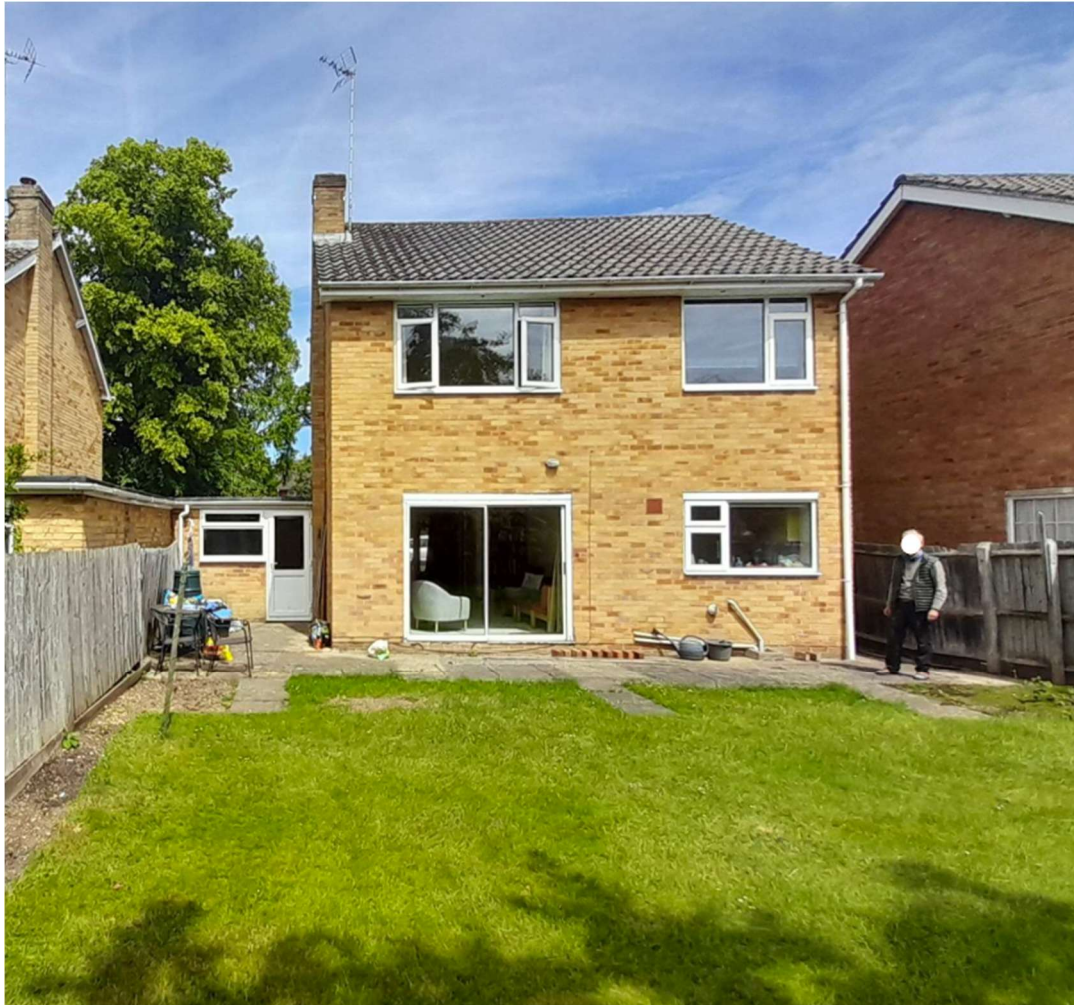
Looking towards the existing rear elevation
