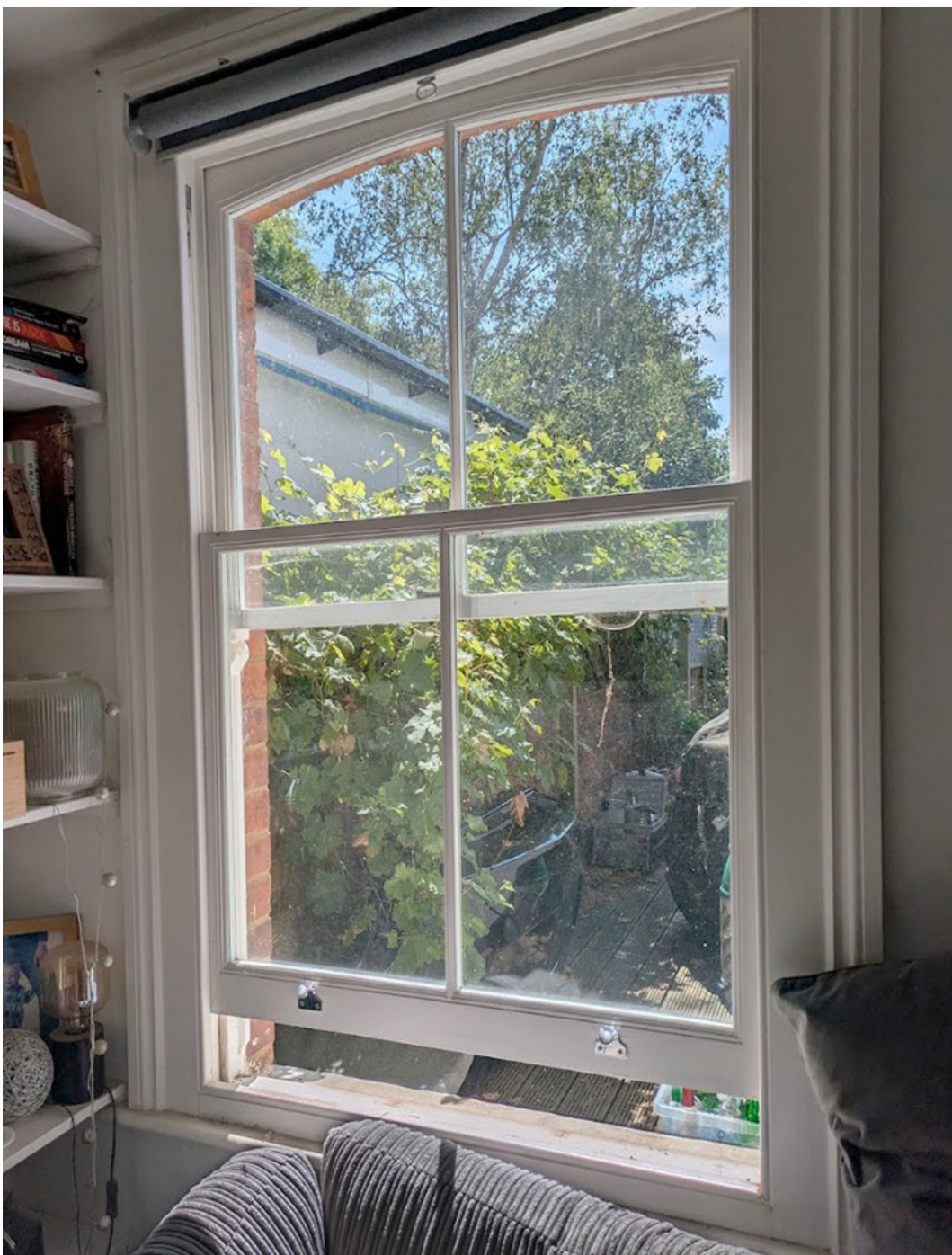
Figure 8: Photo taken from Number 8 School Terrace showing how the extension at number 7 appears. This extension is almost identical to the one proposed for number 5.
