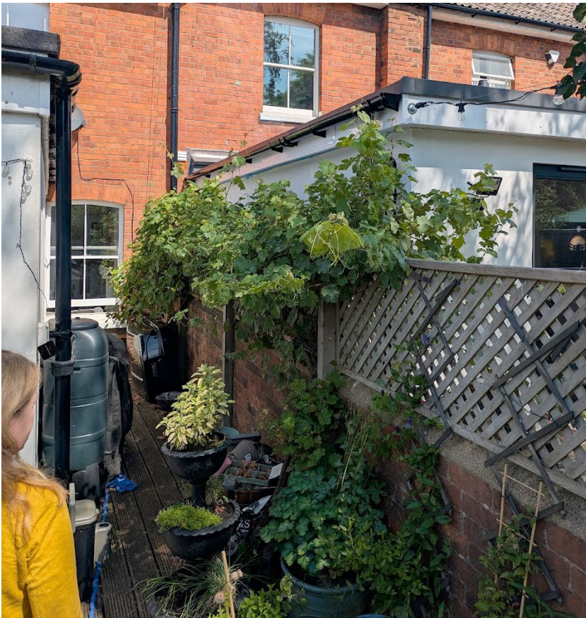
Figure 22 : View of number 7's extension from the garden of number 8.
