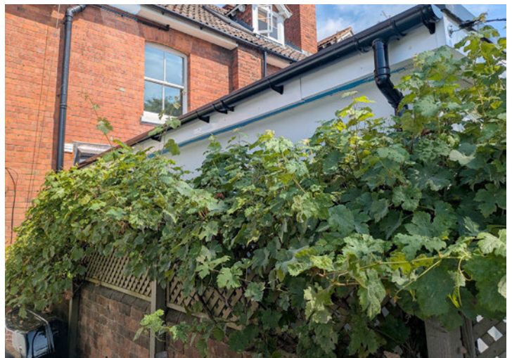
Figure 9 : View of number 7's extension from the garden of number 8.
