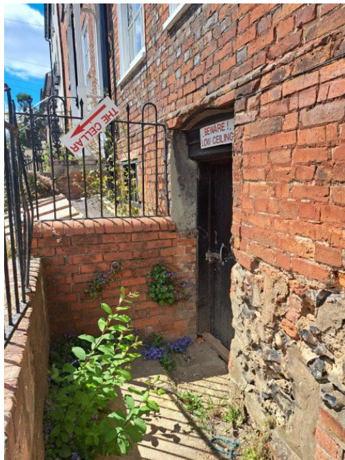
Photo 10-12 – View of front garden and entrance to basement (north elevation)
