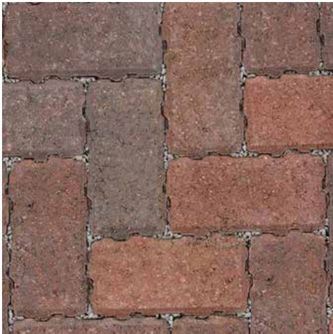
Hard standing areas - Marshalls Priora Driveway Block Paving Brindle (permeable)
