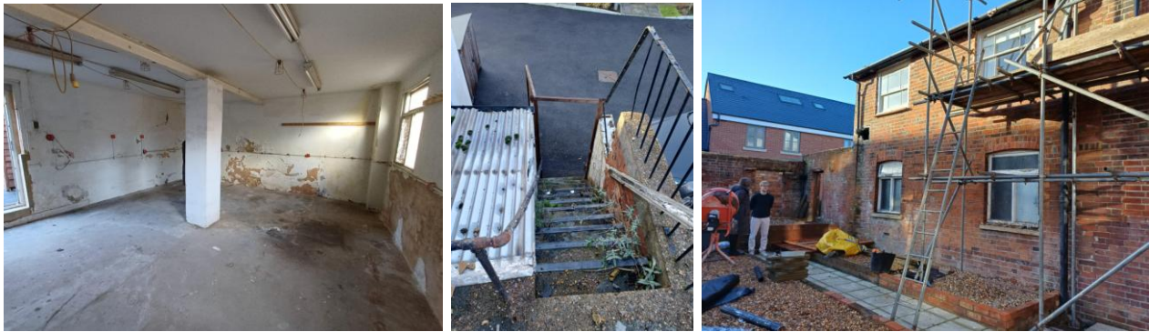
Site visit photos 19/12/2025 – ground floor (left), external stair (centre) & east elevation (right).
