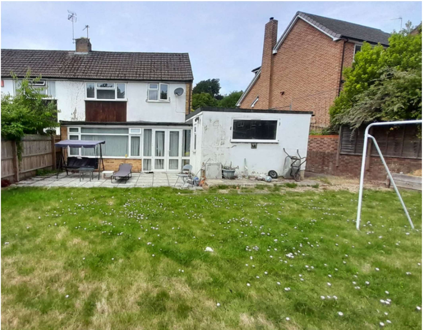
Looking westerly towards existing rear elevation with current single storey extension
