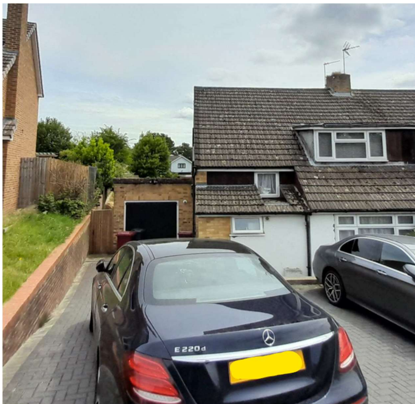
Looking easterly towards front elevation
