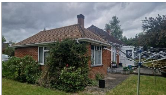
Southern and eastern elevations of B03
