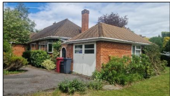
Western and southern elevations of B03
