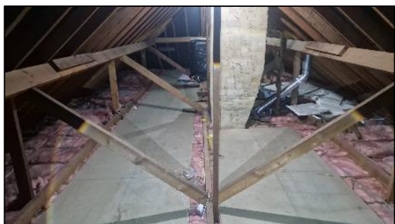
Overview of loft space
