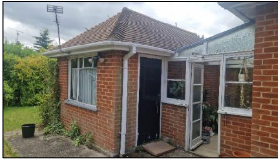
Eastern elevation of B02 and garage (B03)
