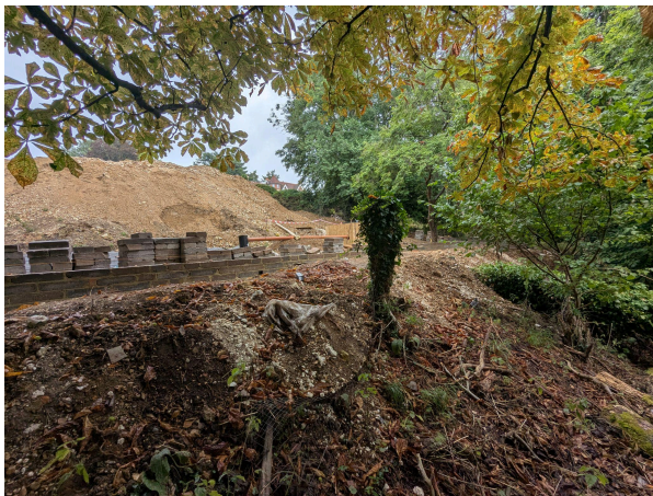
9: Wall construction at southern edge of garden
