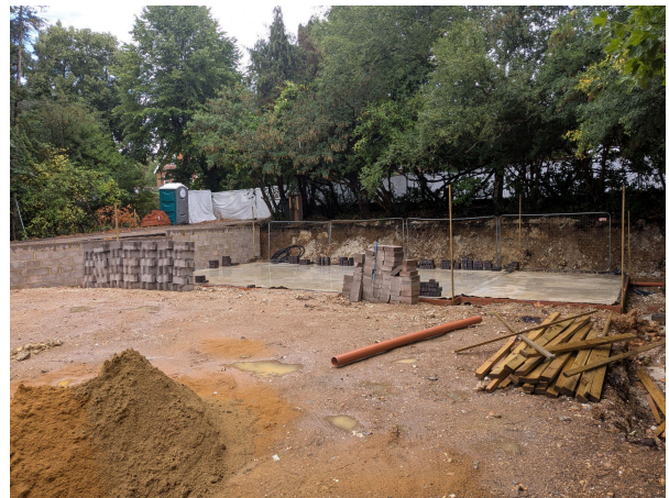
10: Active works area between derelict house and Upper Warren Avenue
