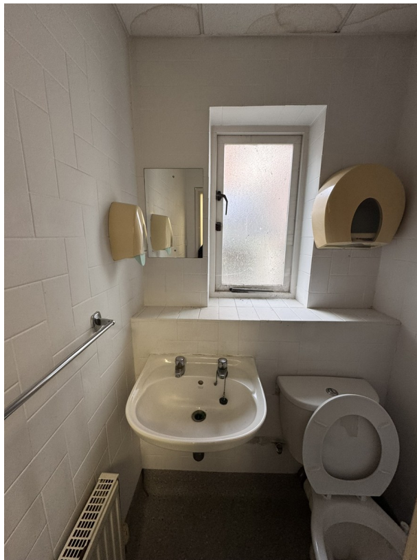
Fig 15—WC F3 in modern rear range
