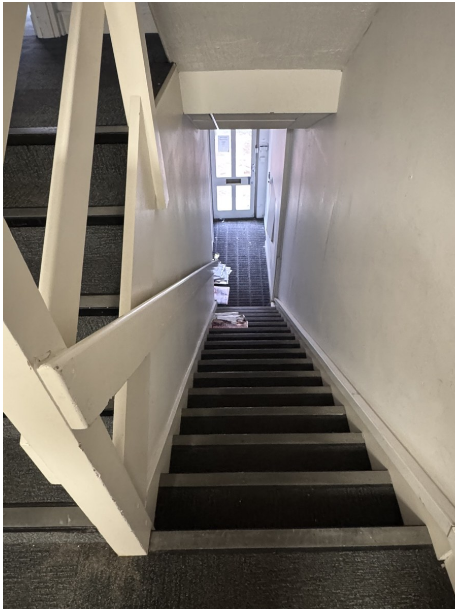
Fig 10—View to Ground Floor entrance hall G1
