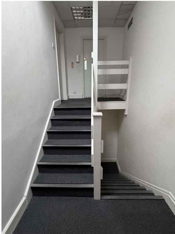
Fig 19—Stair S8 from 2nd floor modern range to 2nd floor historic building
