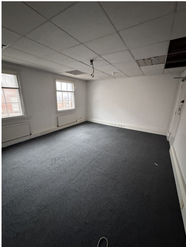
Fig 16—Office S1, 2nd Floor of historic building
