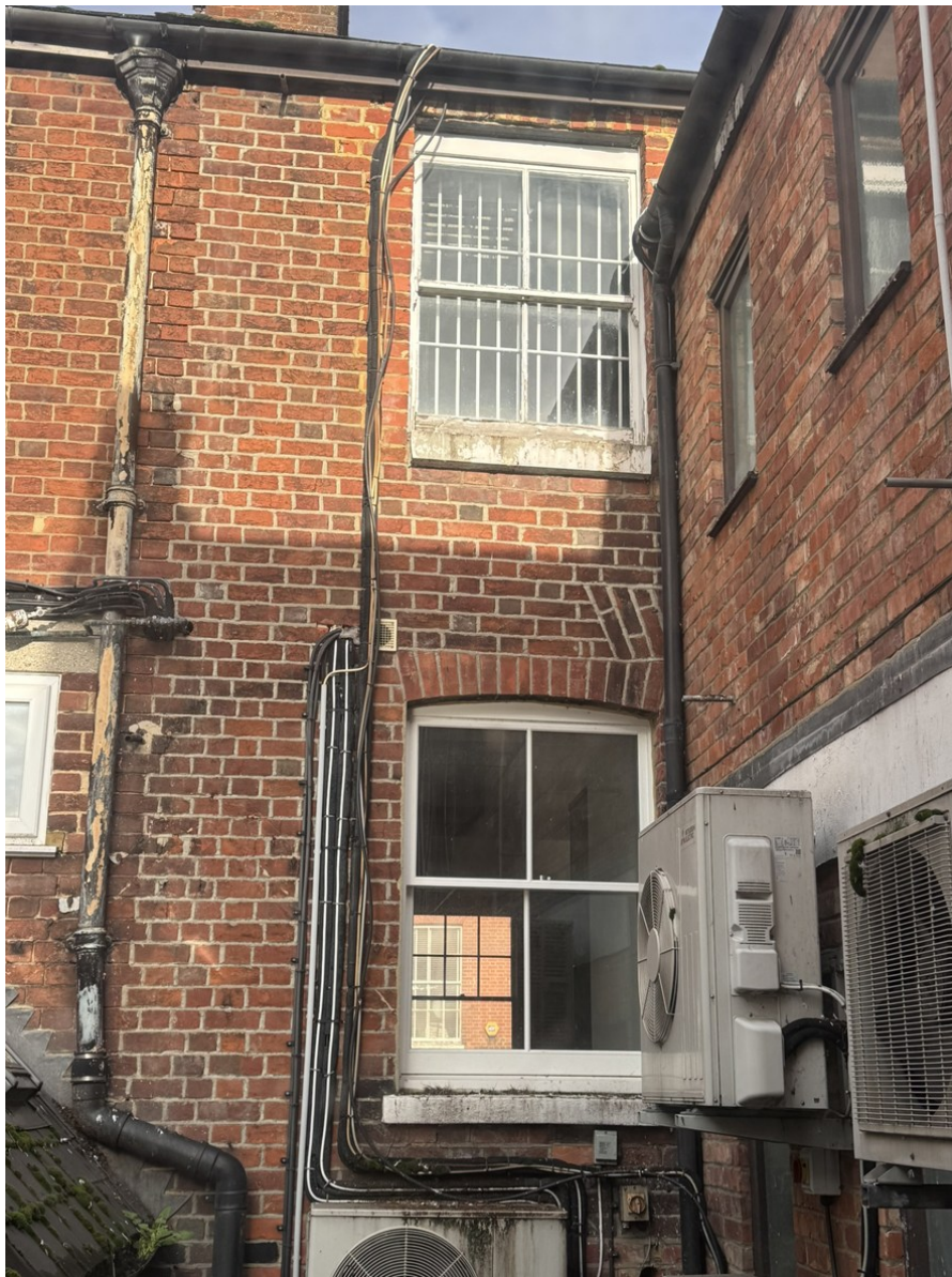
Fig 8—View from 1st Floor of modern range into lightwell and towards rear of historic building
