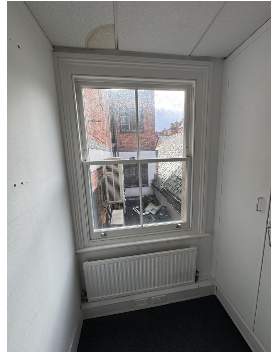
Fig 12—View from room F1 into lightwell
