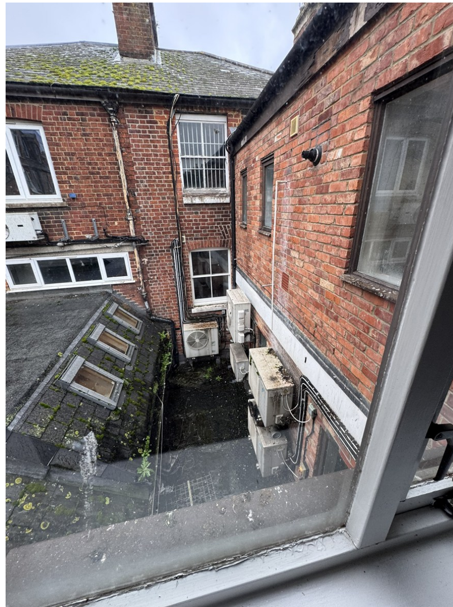
Fig 9—View from 2nd Floor of modern range into lightwell and towards rear of historic building
