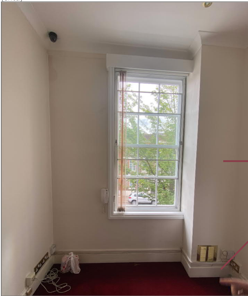
Image 39: First Floor rear northeast room
