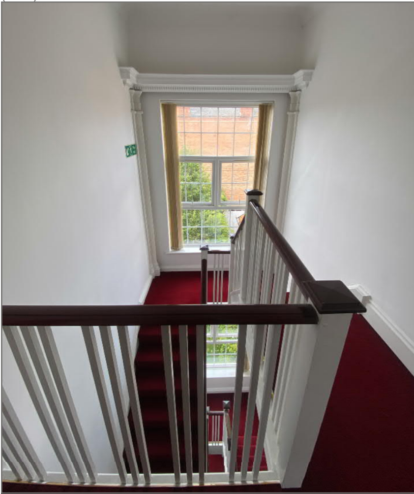
Image 41: View from Second Floor of staircase and window
