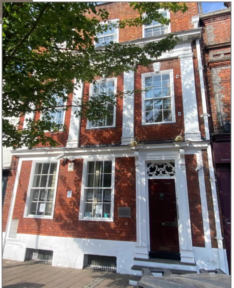
Image 17: View of south elevation and roofline
