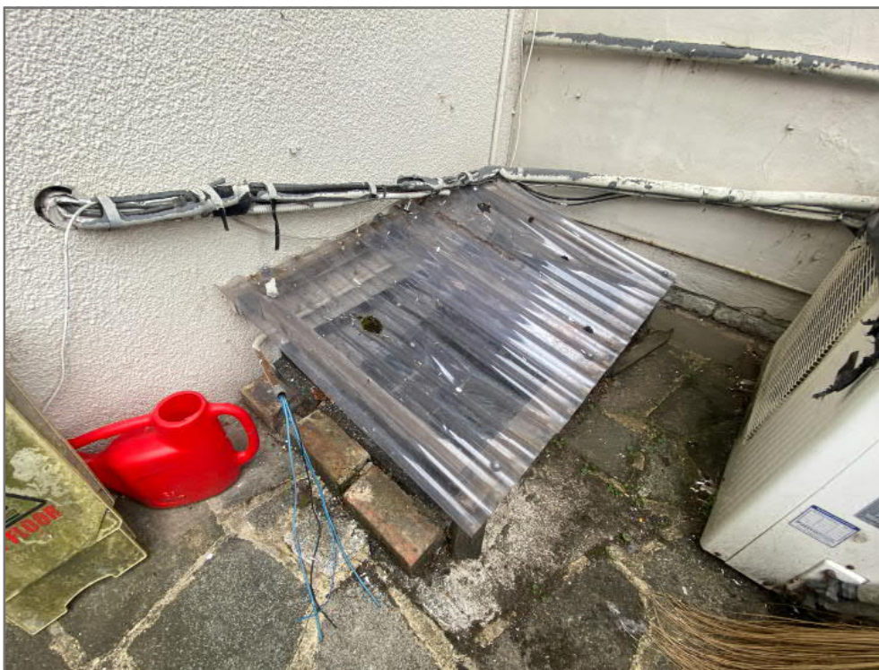
Image 34: Basement window 'W2' protected from water ingress
