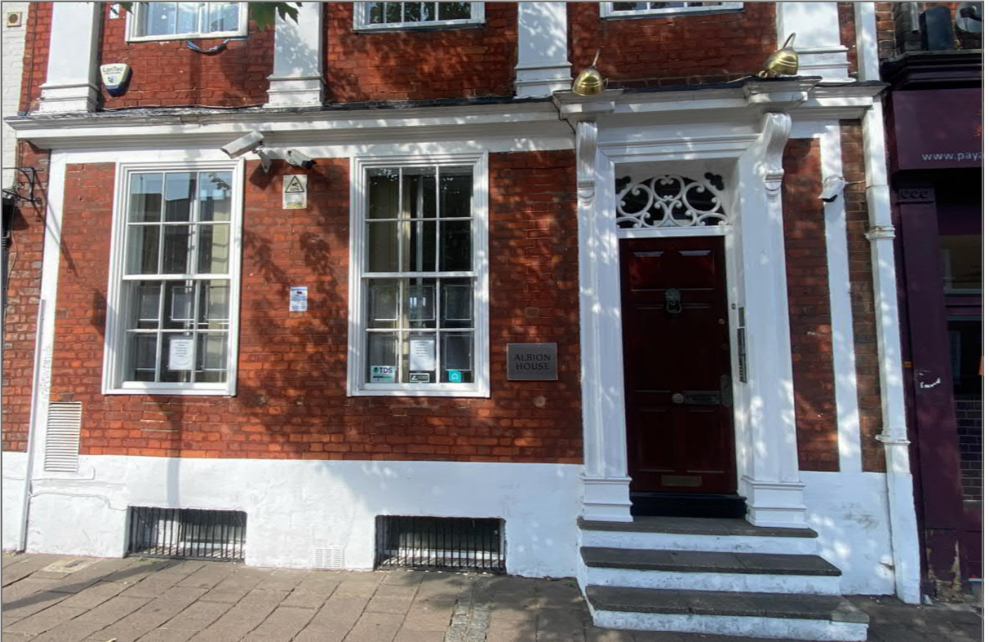
Image 19: Ground Floor detail of east elevation
