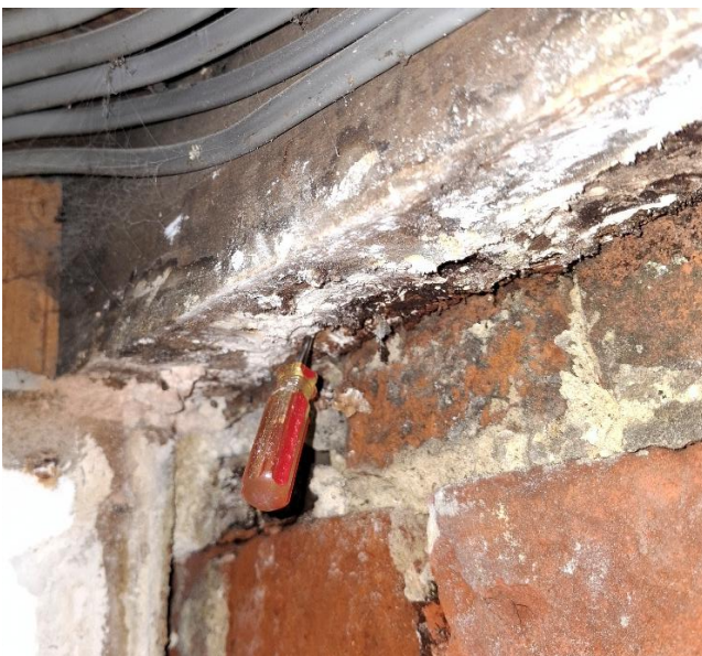
Figure 12. View of timber joist parallel to front elevation basement wall with screwdriver probe
