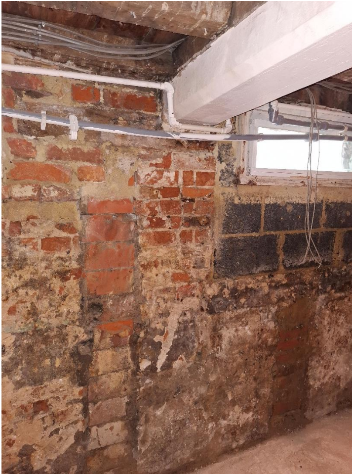
Figure 10. Timber beam supported by remodelled basement wall to the front elevation
