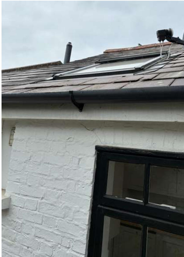
Velux Rooflight within existing roof
