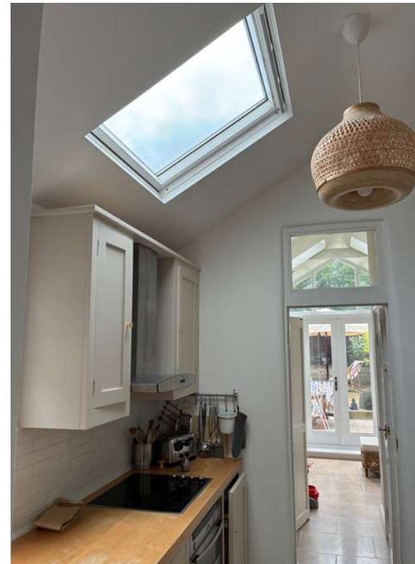
Internal View Rooflight within existing sloping ceiling
