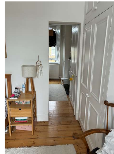
New opening formed into Nursery–Dressing Area
