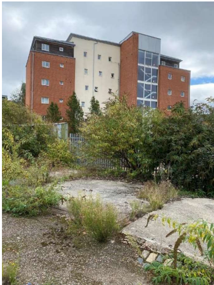
Southern site boundary
