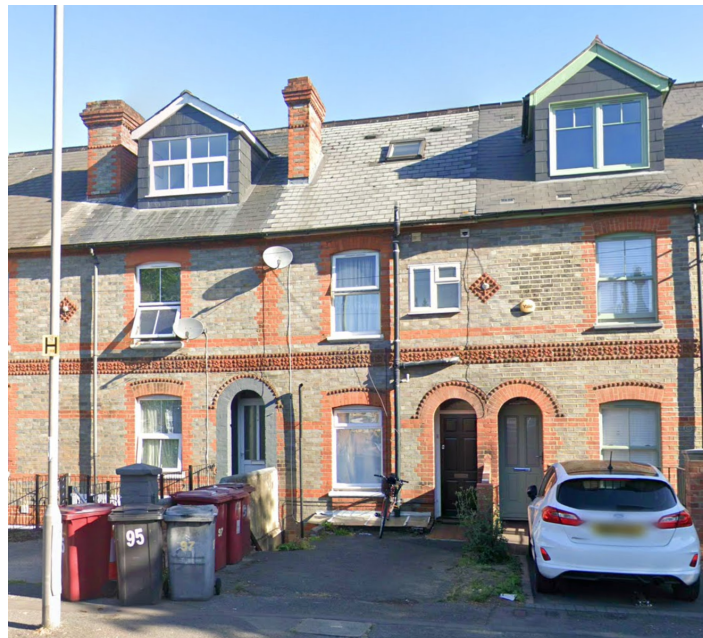
Fig.1: Photograph of 97 Addington Road from the street.
