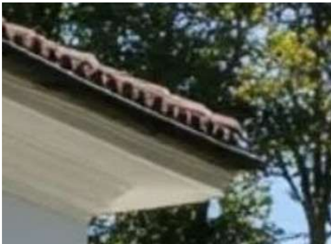
Typical Fascia and Soffit Detail
