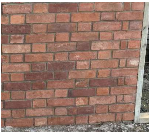
Flemish Bond Face Brick External Walls.
