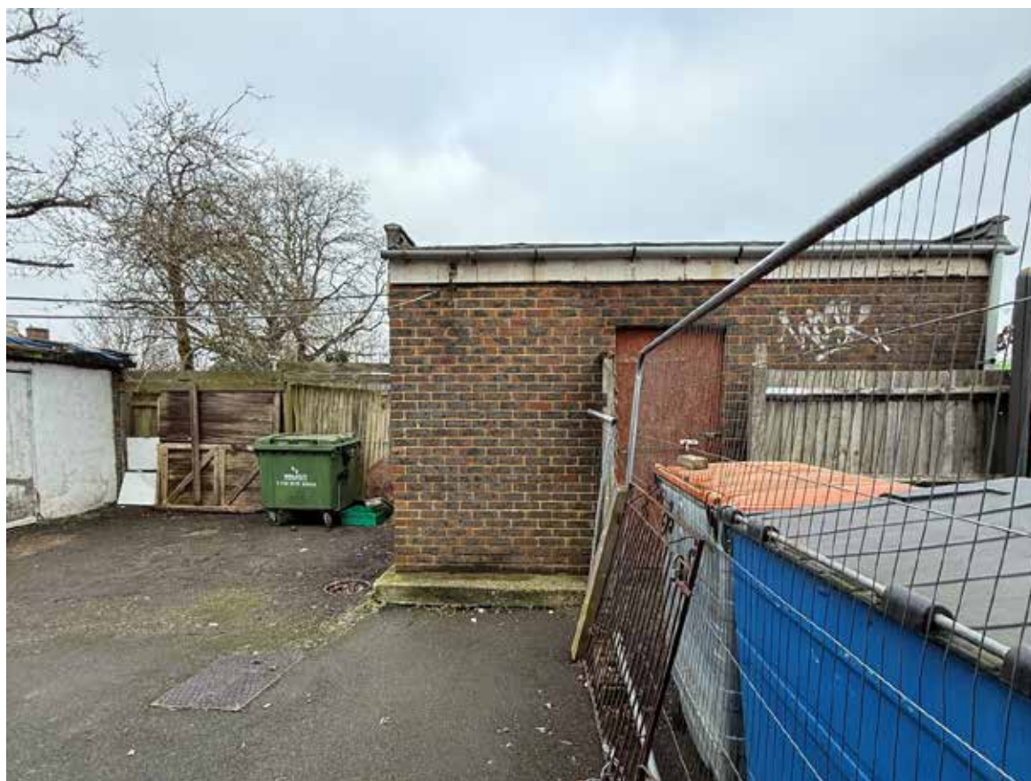
View from rear access yard to shops
