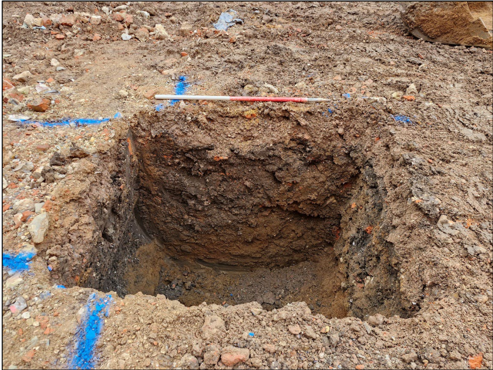
Plate 13: Trench 7, west facing section. 1m scale
