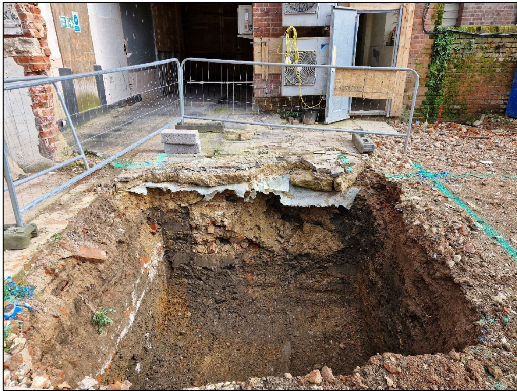
Plate 5: West facing section, Trench 3.
