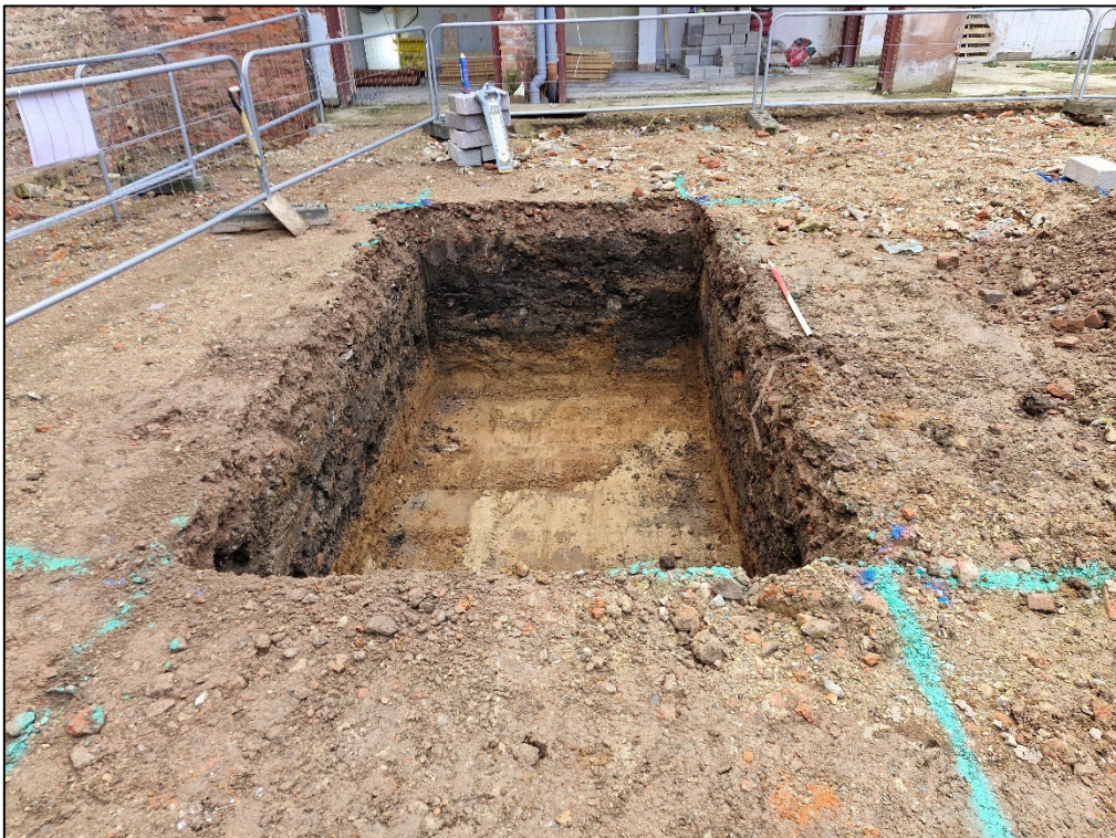
Plate 2: Trench 1 after excavation. View to the south. 1m scale
