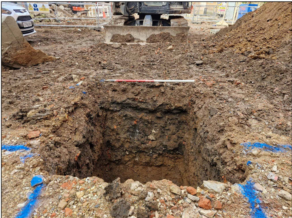
Plate 14: Trench 7, north facing section. 1m scale
