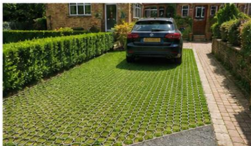
Figure 3: Example of Reinforced Grass Driveway in Use
