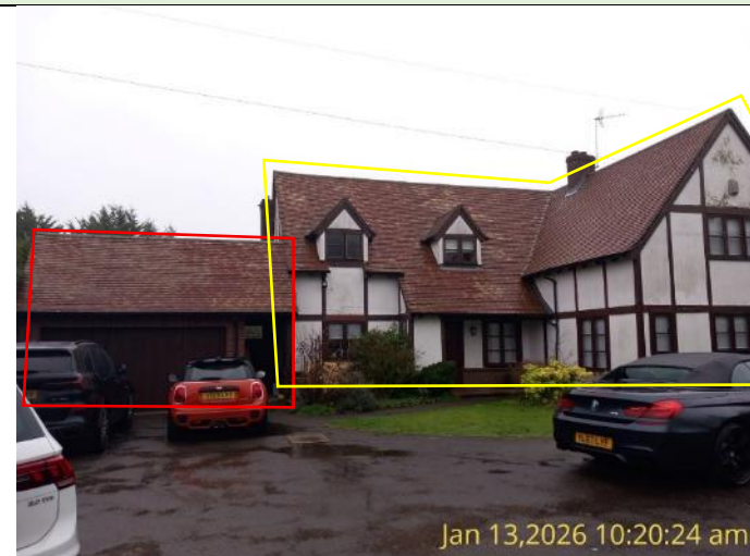
Figure 1: B1 – Northwest elevation.
