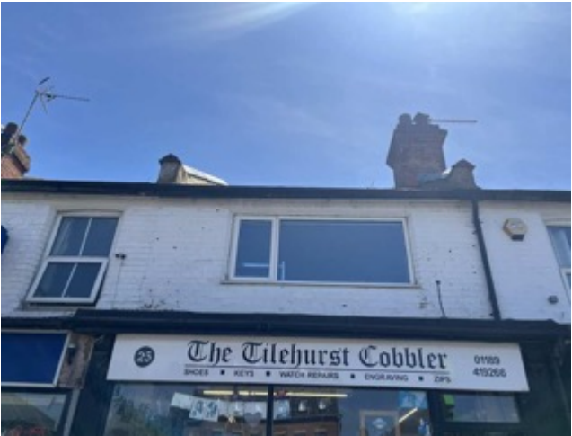
Building B1, northwestern elevation
