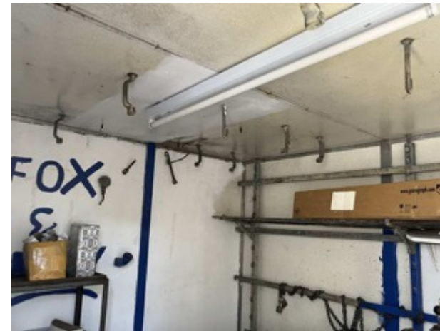
B2 internal void, facing northeast
