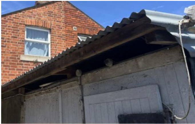
Building B2, southwestern elevation
