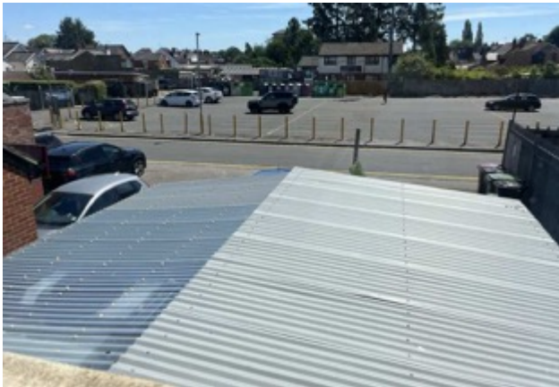
Building B2, corrugated iron roof
