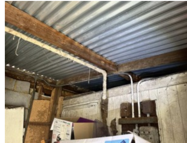
B2 internal void, facing north
