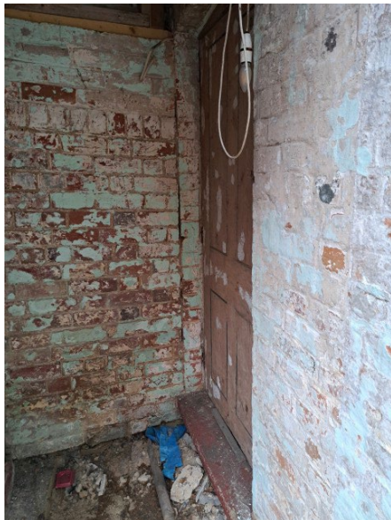
Photo 31 – View the rear exit (?)
