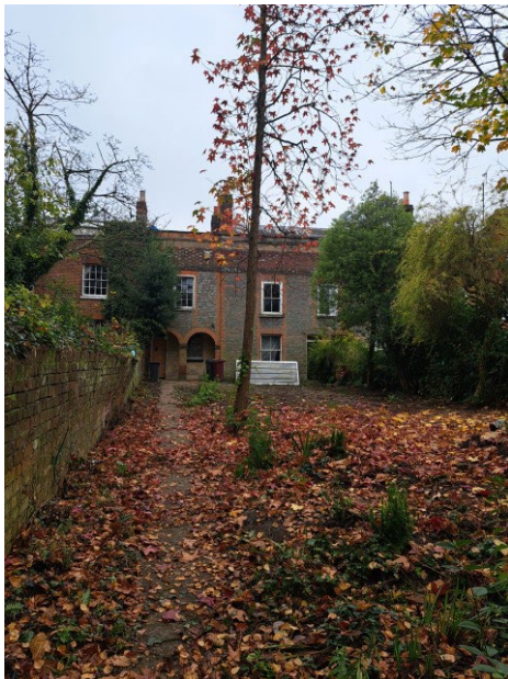
Photo 2-4 – View of front elevation
