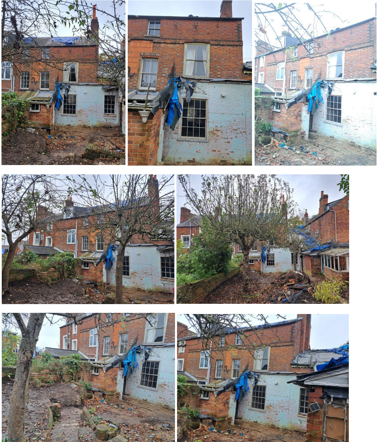
Photo 20-26 – View of the rear elevation (southwest elevation)
