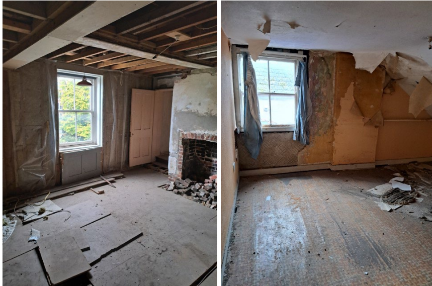
Photo 15 and 16 – View of the interior on the second floor (?)
