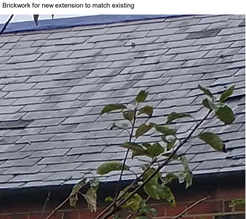
Slate roof to new extension
