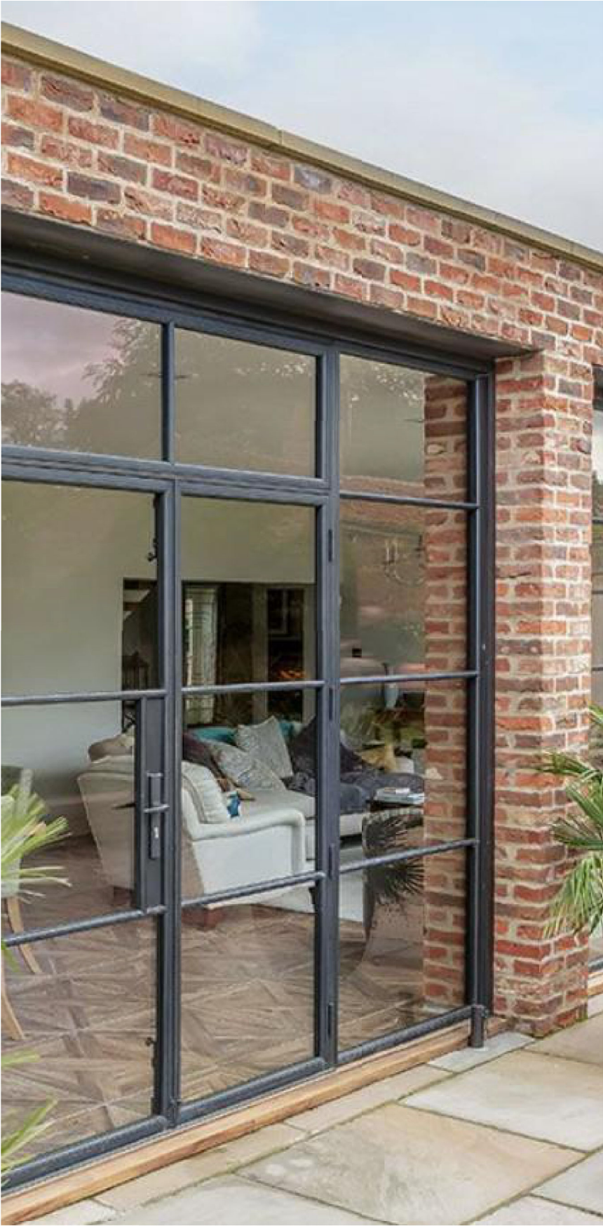
Red brick and Crittall glazed framing to new extension
