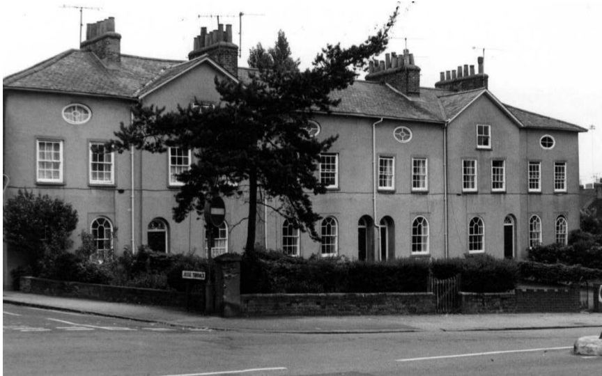
Photograph of listed 134-144 (even) Castle Hill, September 1981
