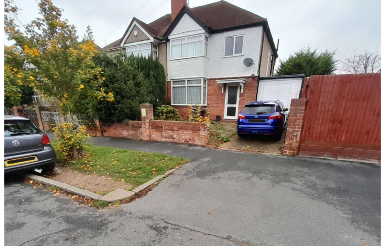
Site visit – Existing Front Elevation
