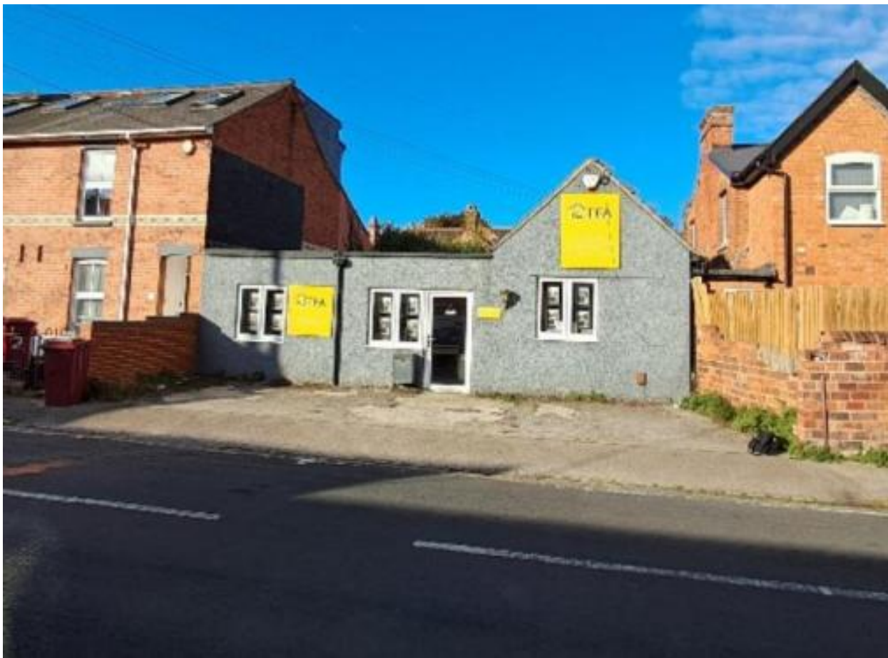
Figure 1: An image of the entrance to Mandeville Courtyards as accessed from Warriner Gardens to the north.
