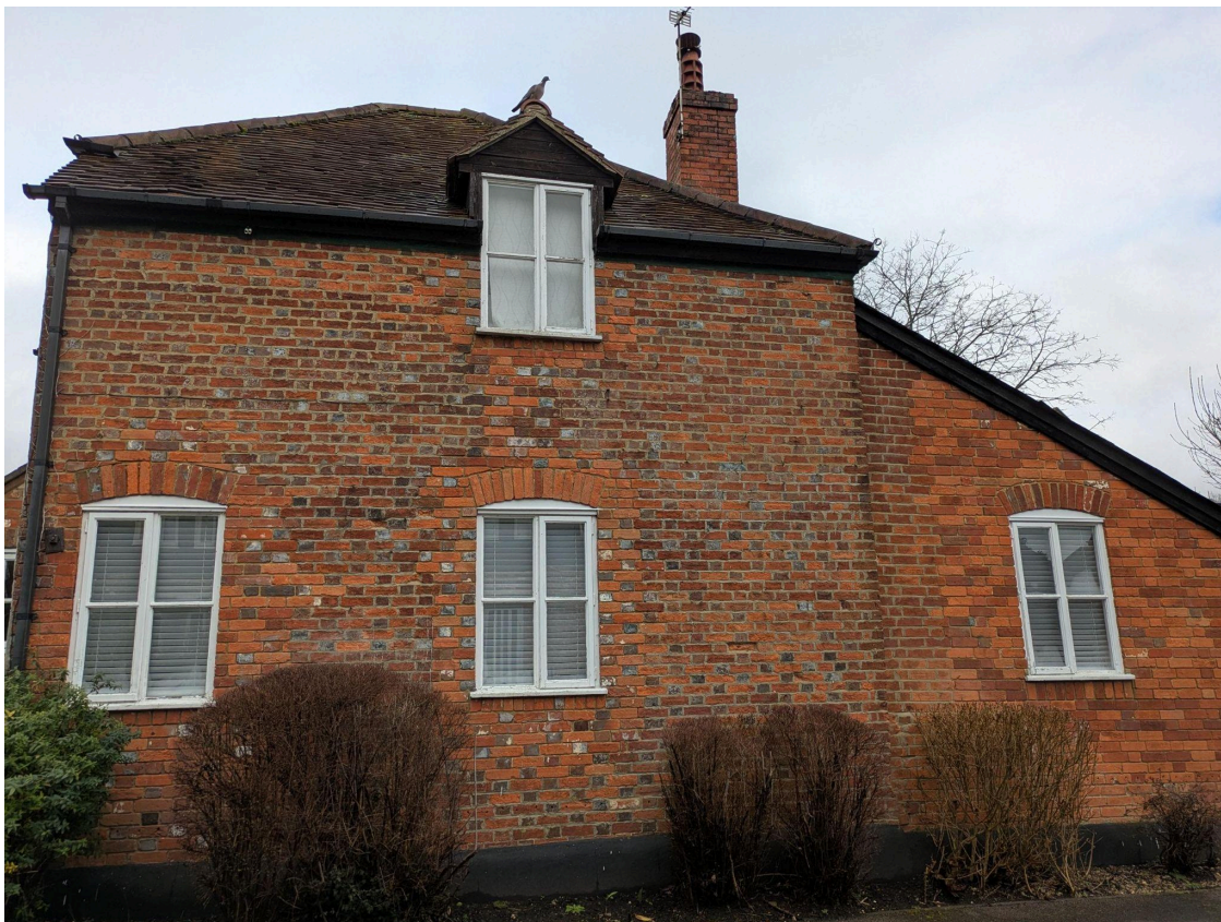
Above. Rose Cottage, 1 Yew Lane, showing the existing casement windows each with one opening and 1 fixed casement.
