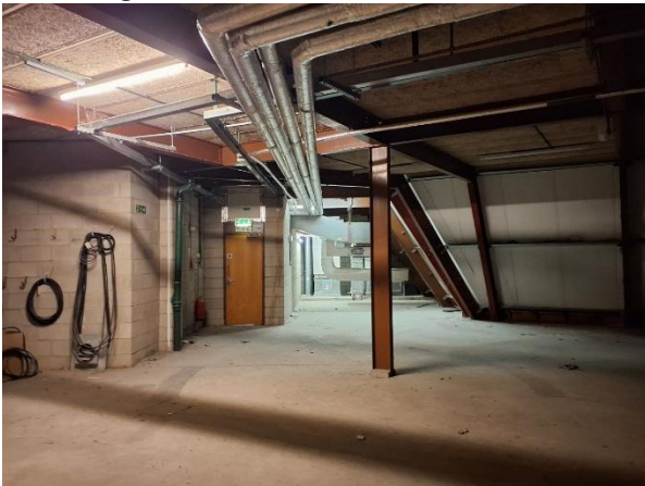
7. Reading Police Station interior.
