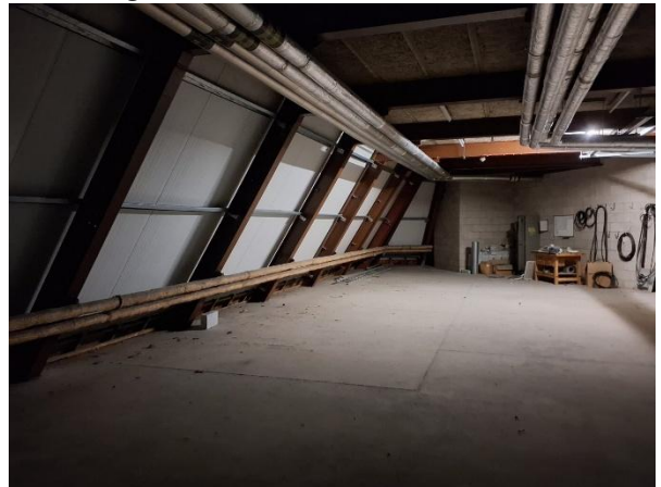
6. Reading Police Station interior.
