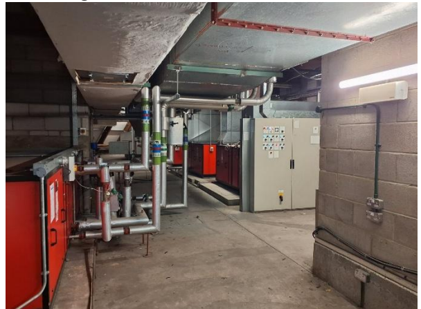
8. Reading Police Station interior.
