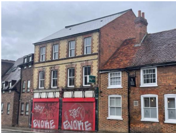
South-eastern and south-western elevations
