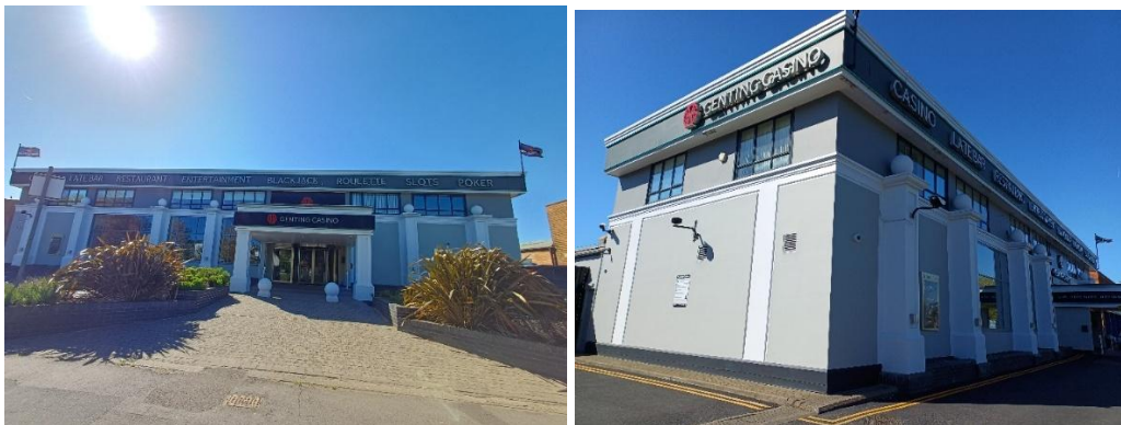
Front & east side views of 18 Richfield Avenue, taken on 29/04 & 10/04/26 respectively by the Officer
