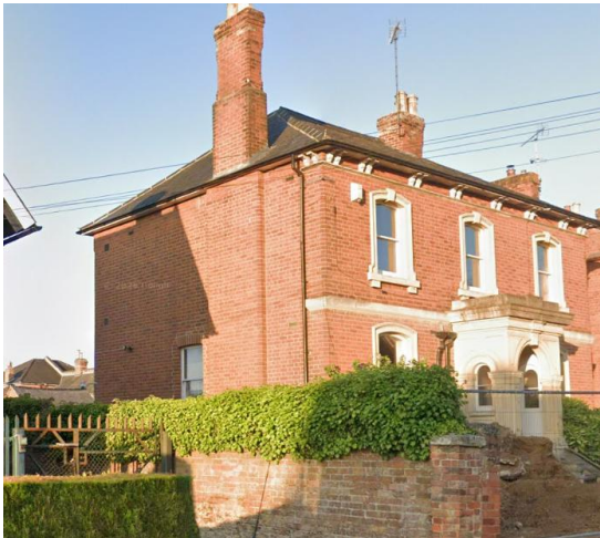
Side facing no. 83 Hamilton Road (one existing gf window)
