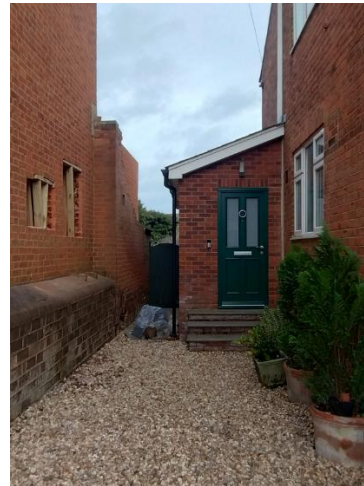
Side facing no. 87A Hamilton Road (two new window openings partially constructed)
