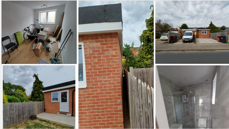
Figure 2 - Site Visit Photographs
