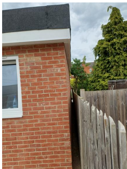
Figure 4 - Site Photo showing building relative to side boundary
