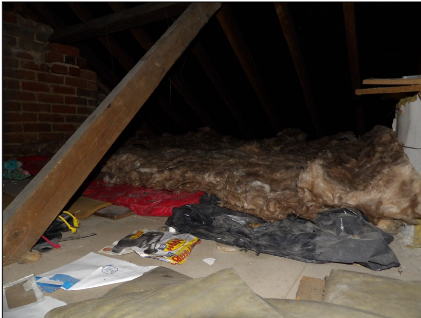
Figure 10. Example loft space and bitumen felt lining to tiles. 101 Belmont Road, Reading. 16.06.26
