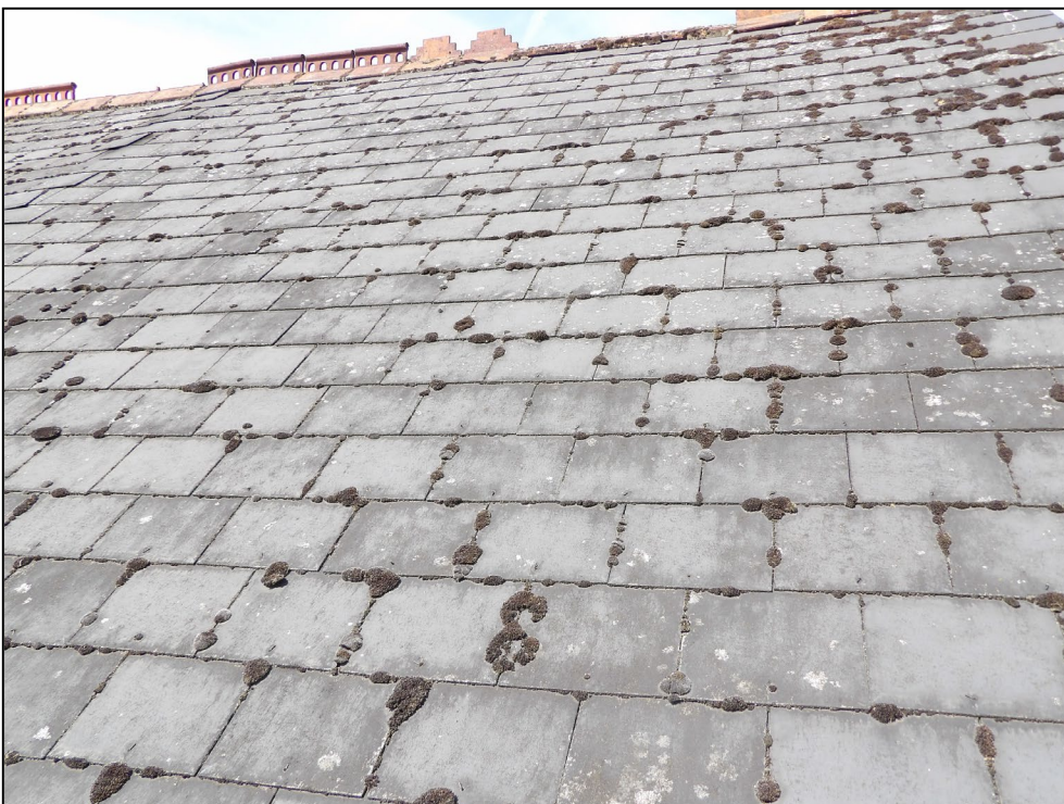
Figure 5. Example slate covering on roof. 101 Belmont Road, Reading. 16.06.26
