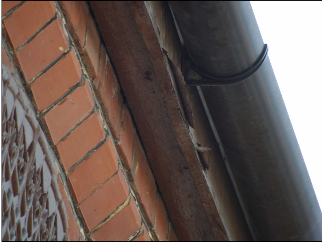
Figure 8. Example well fitted soffits and fascias. 101 Belmont Road, Reading. 16.06.26
