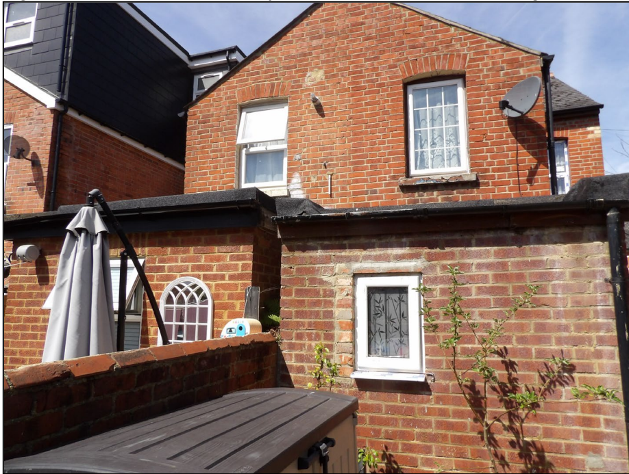
Figure 4. Rear view of property. 101 Belmont Road, Reading. 16.06.26
