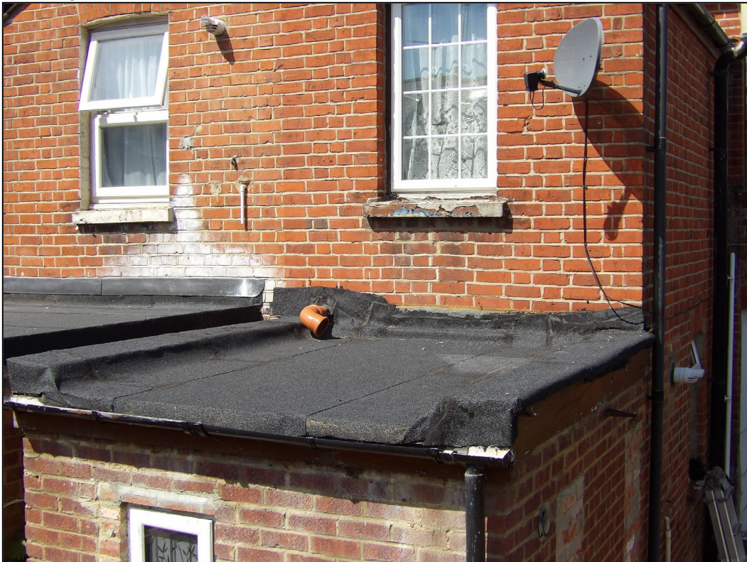
Figure 9. Bitumen covering rear extension and flush fascias. 101 Belmont Road, Reading. 16.06.26
