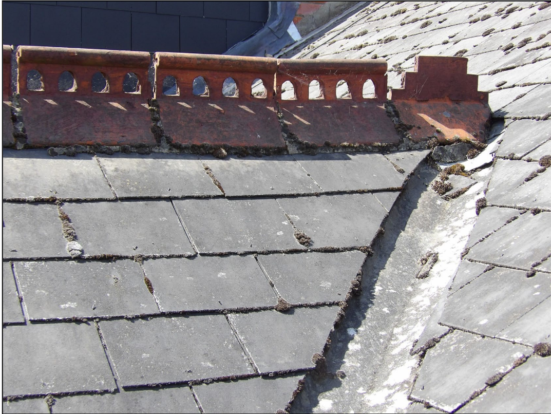
Figure 6. Example sealed ridge tiles. 101 Belmont Road, Reading. 16.06.26
