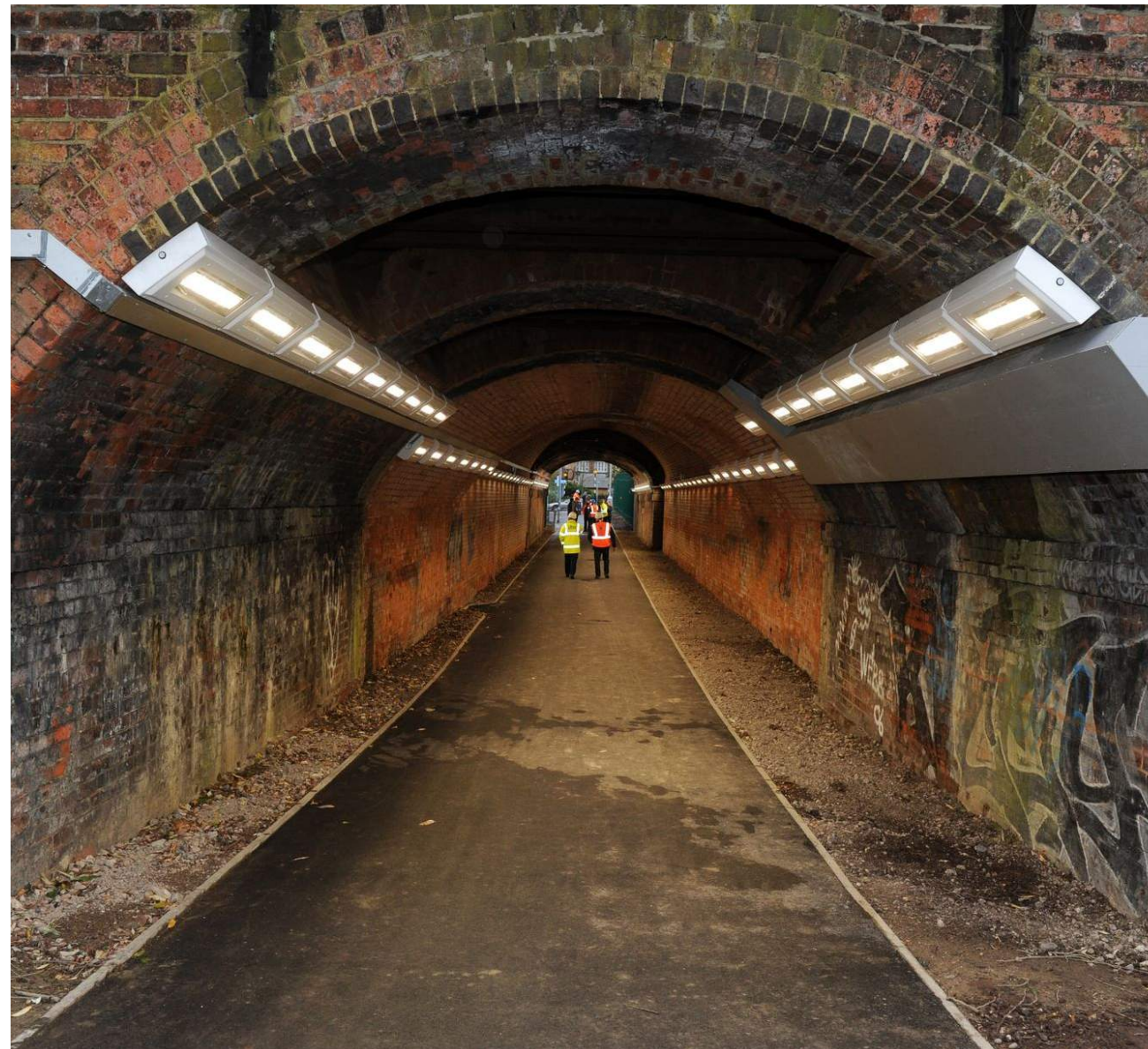
Biscuit Tunnel from Napier Rd to Kenavon Drive
