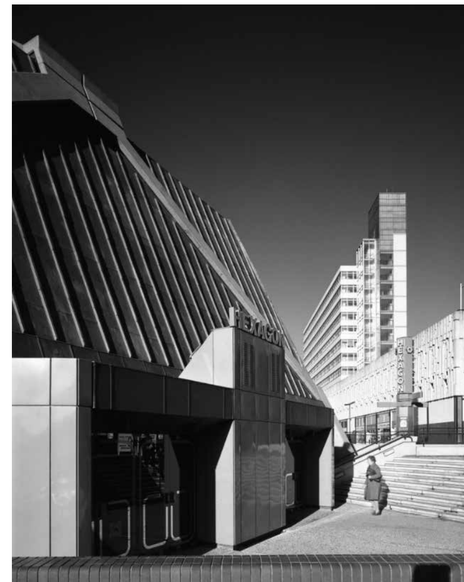
Figure 4.14 View of the Hexagon, Broad Street Shopping Centre and Fountain House, 1979 (RIBA Pix)
