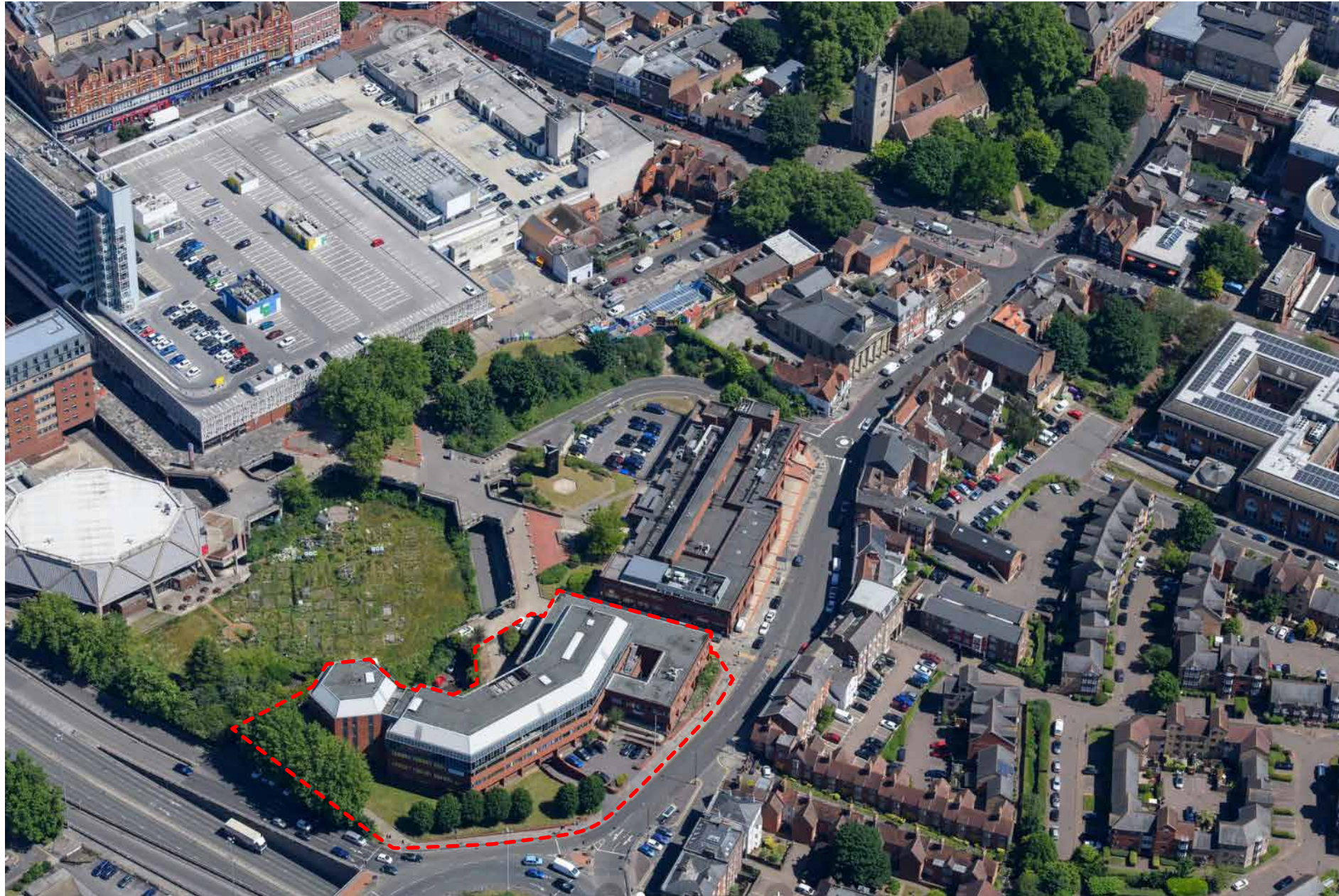
Figure 4.16 Aerial photograph of the Site, Civic Core and Castle Street, showing fragmented townscape in 2022 (Historic England)
