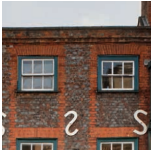
Vertical and soldier brick detailing to group windows
