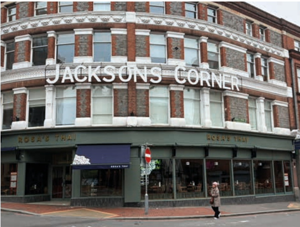
Material changel along the ground floor
