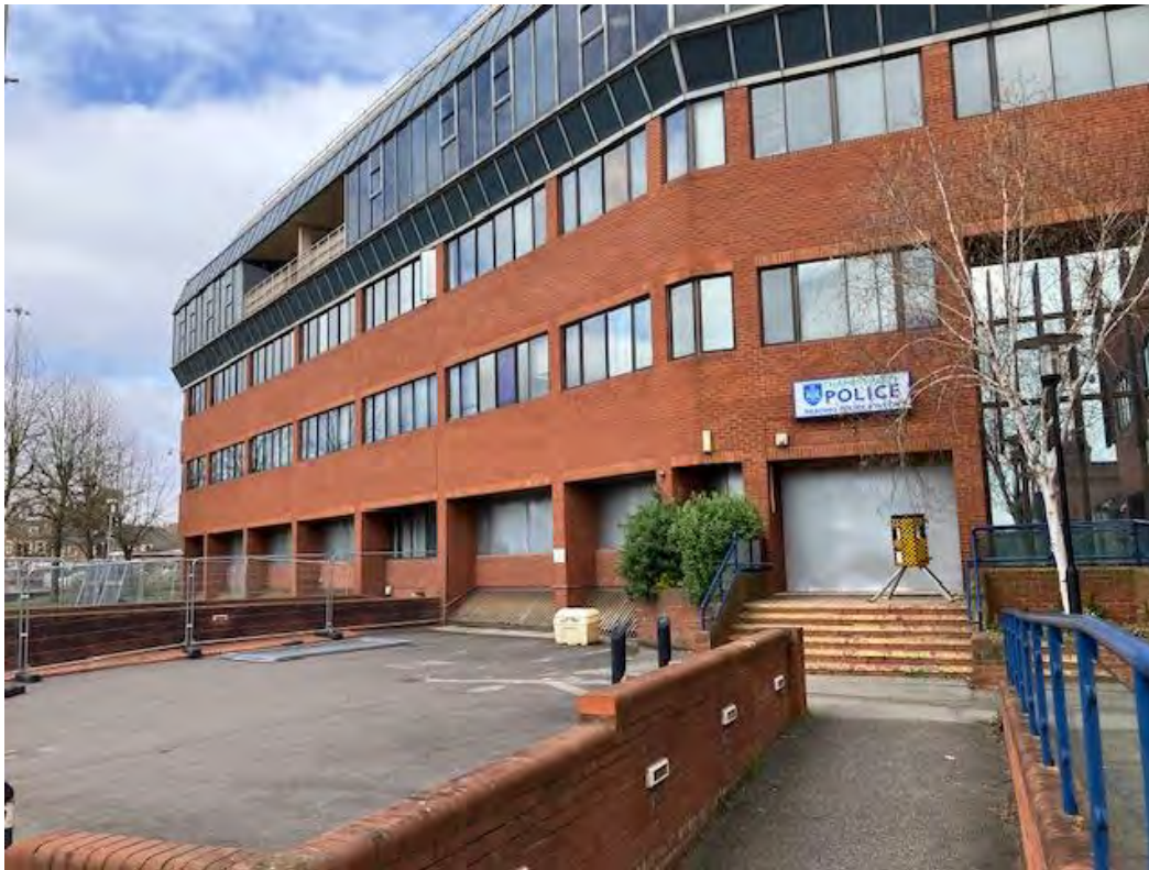
Plate 1: Police Station building and southern yard looking west
