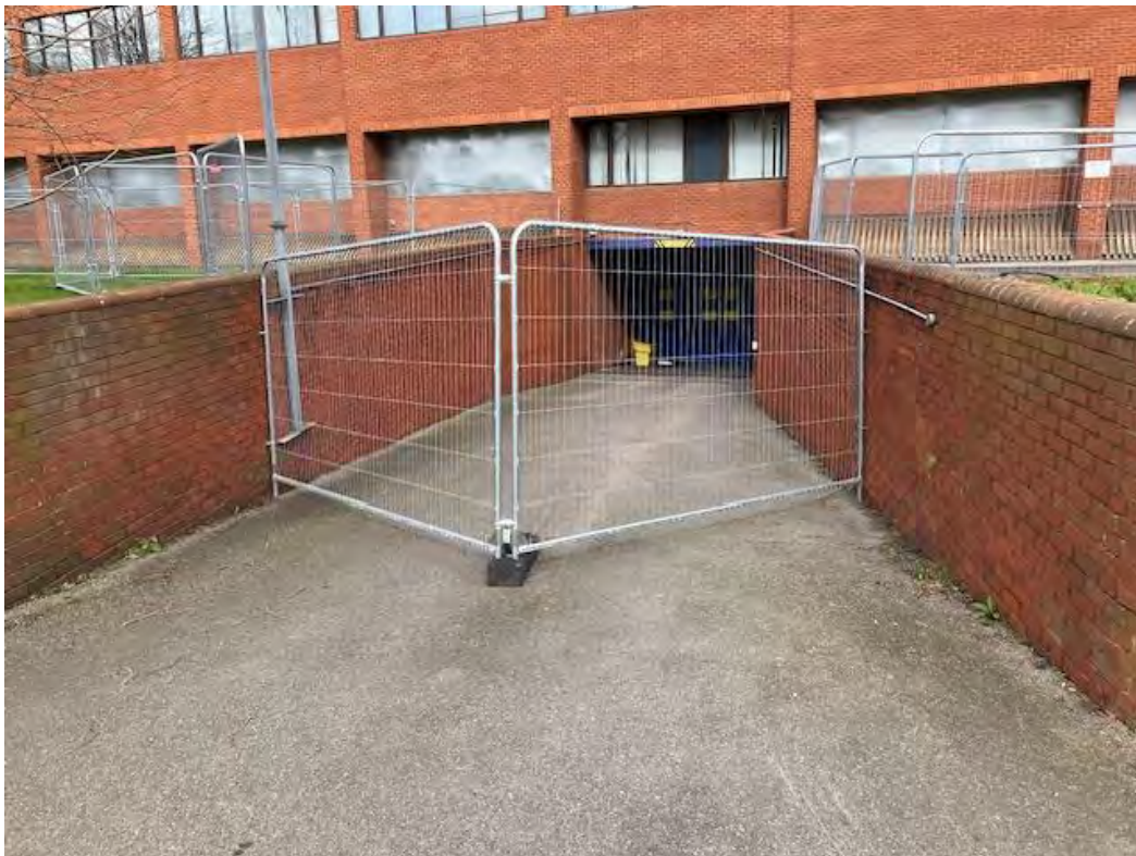
Plate 2: Entrance to basement car park from Castle Road (looking north)
